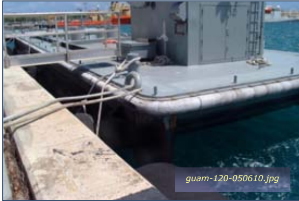
Photo #4-1: SWOB at Victor Wharf Taken By: Greg V. Arthur Date: 05/06/10
