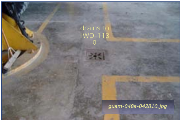
Photo #4-32: Bldg 557C - Example Floor Drain Taken By: Greg V. Arthur Date: 04/28/10
