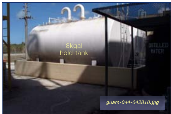
Photo #4-24: Bldg 307 Orote Power Plant – 8K Hold Taken By: Greg V. Arthur Date: 04/28/10
