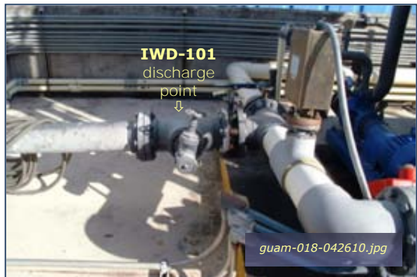
Photo #4-6: Victor Wharf BOWTS – Discharge Point Taken By: Greg V. Arthur Date: 04/26/10
