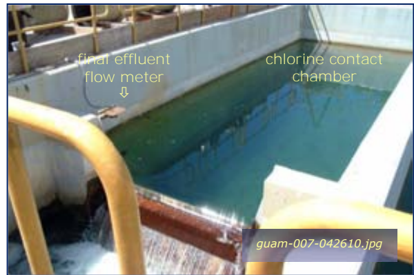
Photo #3-6: Apra Harbor WWTP - NPDES-001 Taken By: Greg V. Arthur Date: 04/26/10
