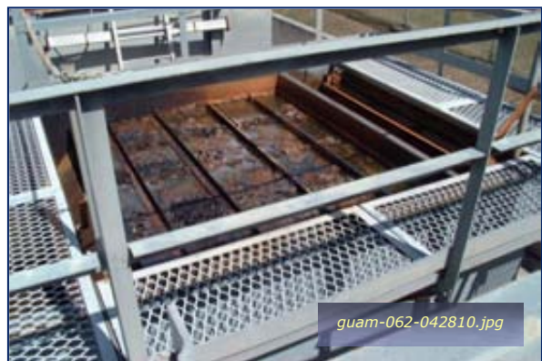
Photo #4-12: FISC Fuel Farm - O/W Plate Coalesce Taken By: Greg V. Arthur Date: 04/28/10
