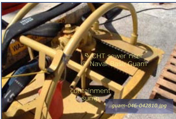
Photo #3-9: Sierra Wharf CHT Sewer Riser Taken By: Greg V. Arthur Date: 04/28/10
