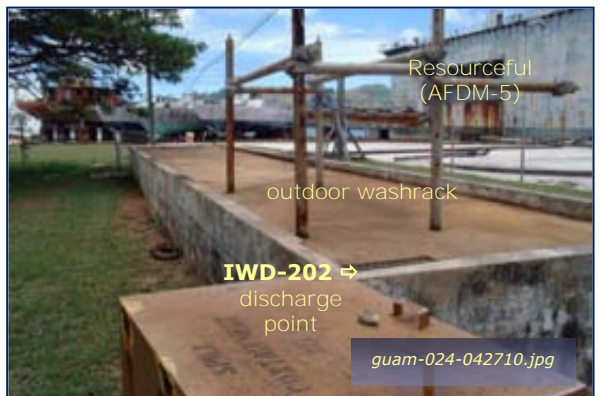
Photo #5-4: Papa Wharf O/W Treatment - Discharge Taken By: Greg V. Arthur Date: 04/27/10
