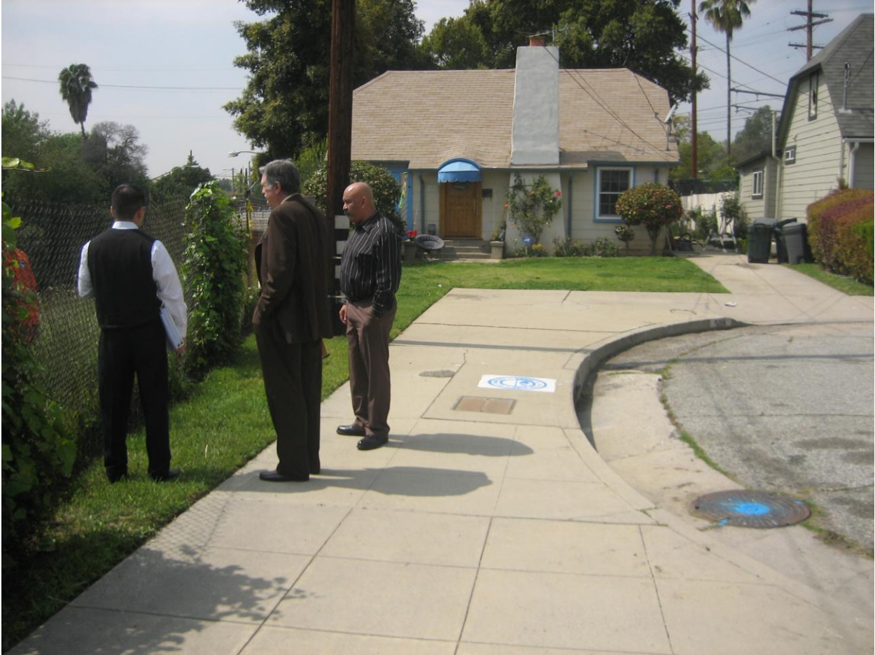
Figure 12: Location of manhole and storm drain inlet at the end of Mound Ave. where it abuts I-110 freeway. City stated that the manhole on opposite side of the fence (see Fig. 11), surcharged but did not overflow.
