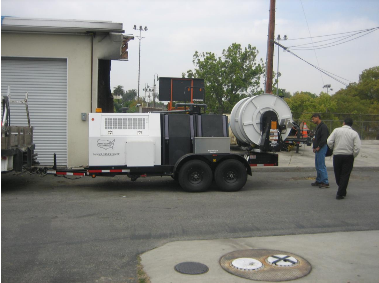
Figure 6: Combination generator/jet rodder/CCTV trailer at city maintenance yard
