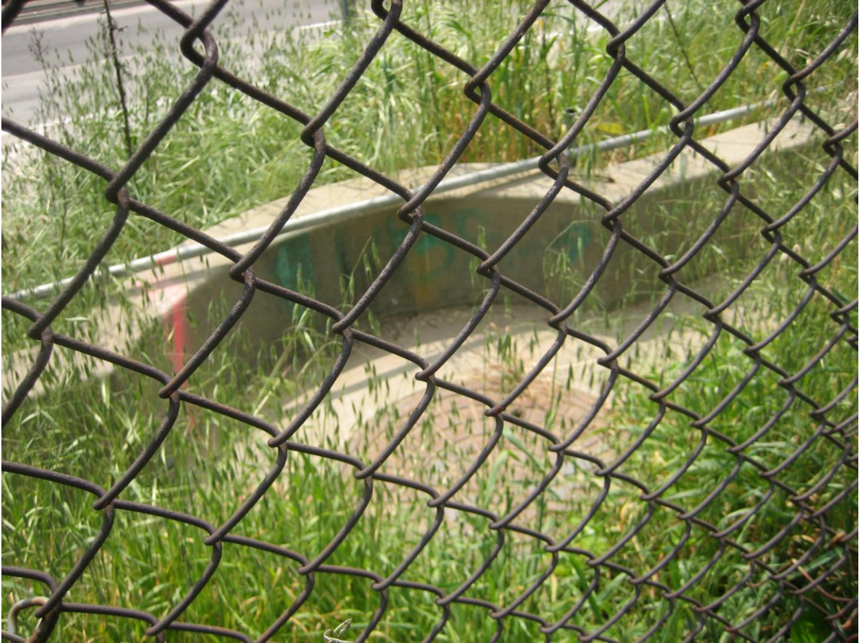
Figure 11: MH143B, the first manhole upstream from the Fair Oaks at State St. spill site, at the end of Mound Ave. This manhole is above the westbound onramp to the I-110 freeway. City staff indicated that this manhole was the first manhole downstream from the root blockage and surcharged but did not overflow.
