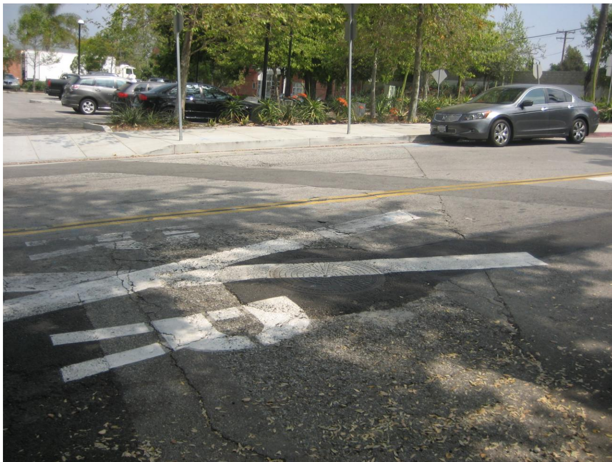
Figure 13: Site of October 10, 2009 spill at 1020 Arroyo Verde Road. City staff explained that this spill was due to a cracked pipe and excessive roots infiltrating main from an unused lateral connection. City staff said that the manhole is shallow, relative to upstream and downstream manholes. Three spills occurred within two weeks at this location, although smaller in volume than the Fair Oaks spill. The lateral connection was later eliminated and a pressure manhole cover installed.
