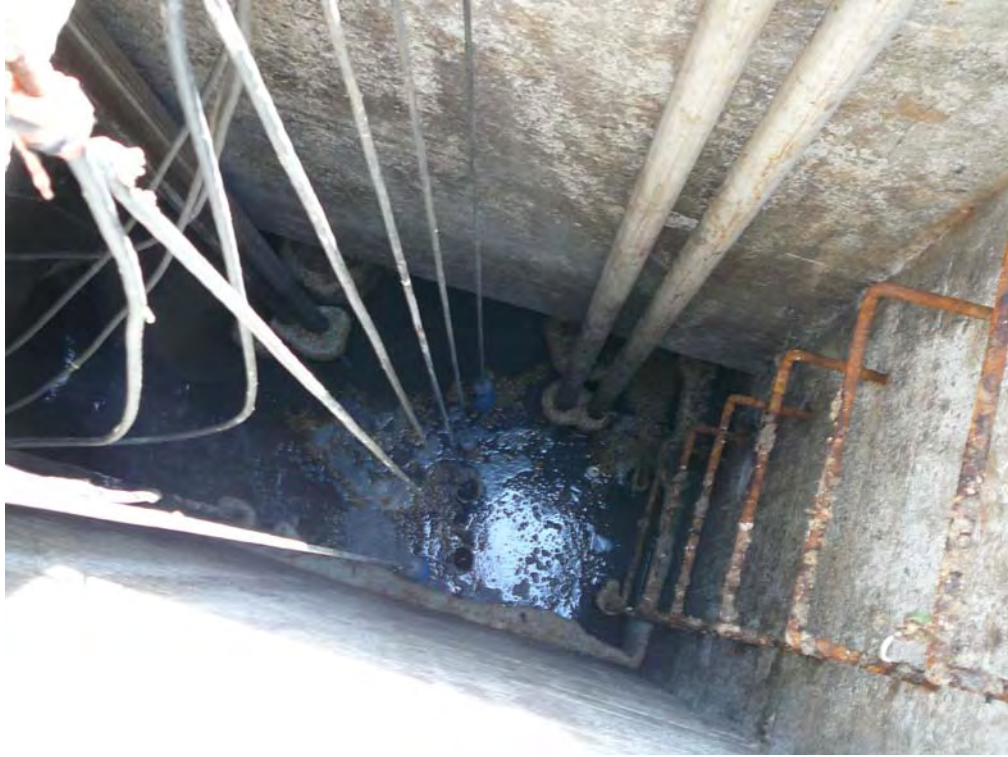
Photo 1 Burlingame pump station wet well
