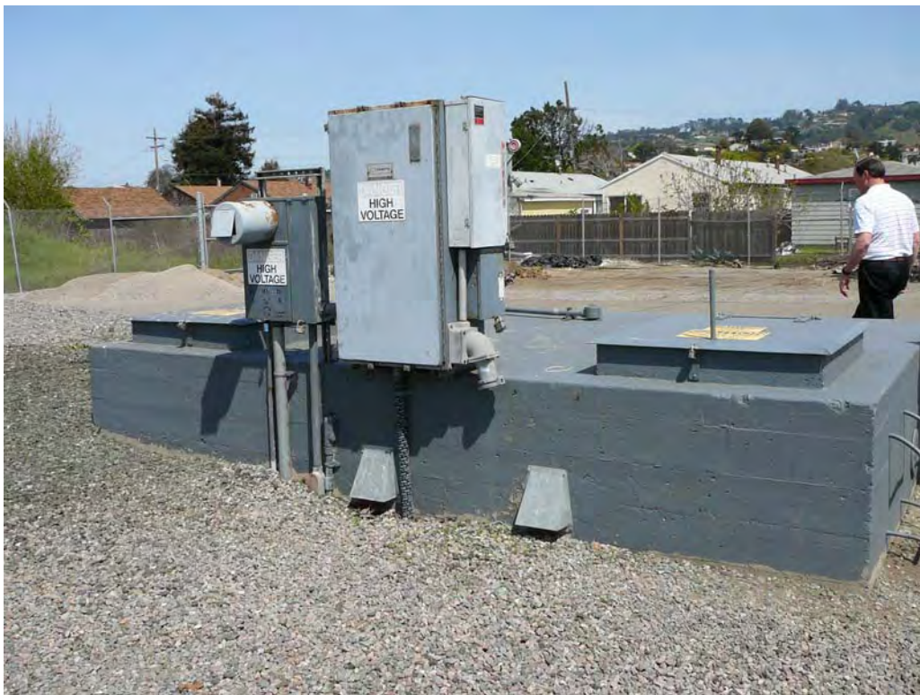
Photo 4 Outside view of Burlingame pump station
