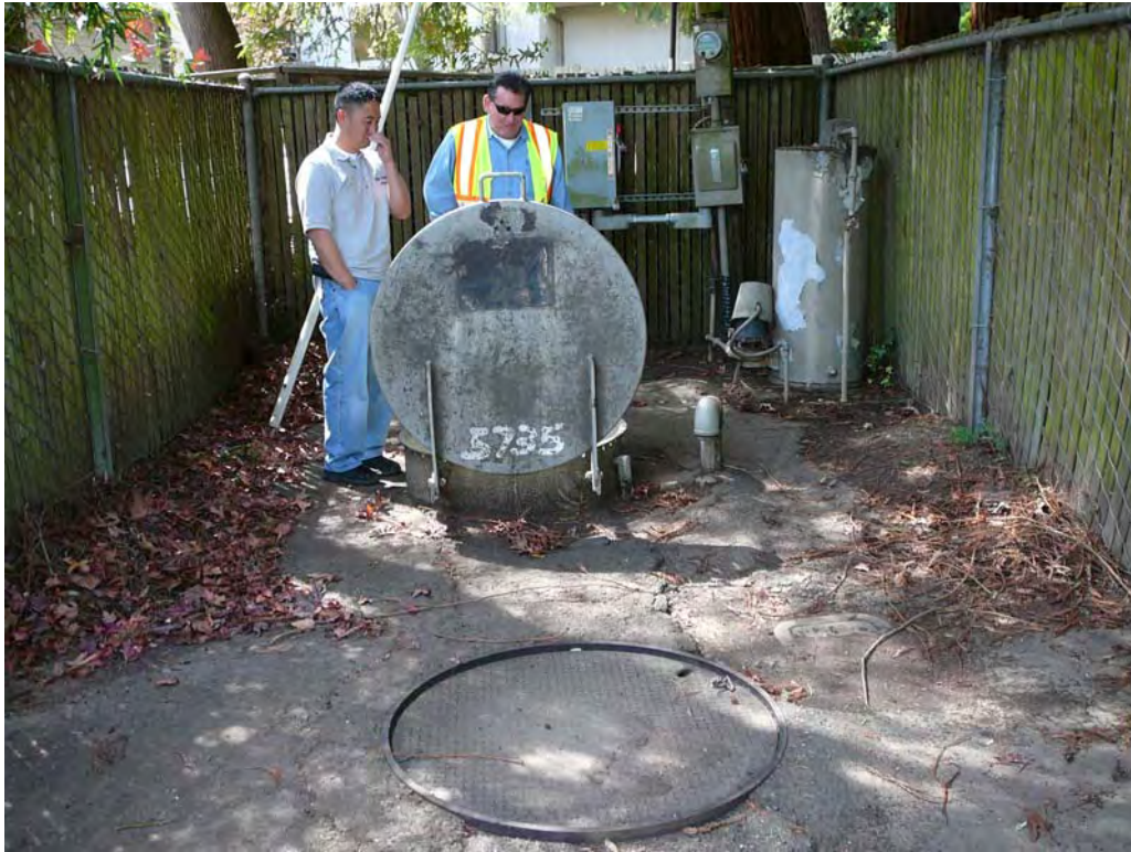
Photo 5 Cannon pump station
