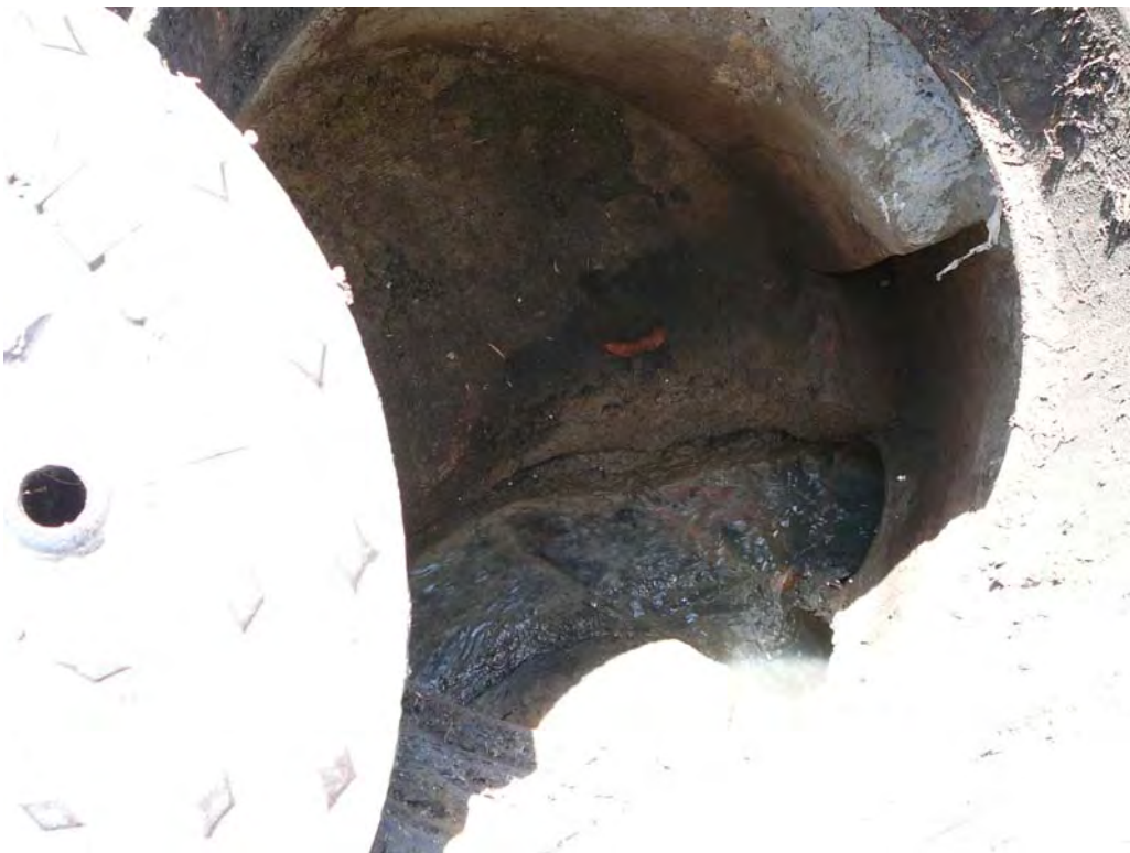
Photo 10 "4 Pomona" - capacity spill site
