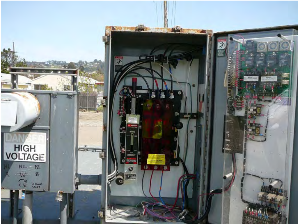
Photo 3 Controller and emergency switch at Burlingame pump station
