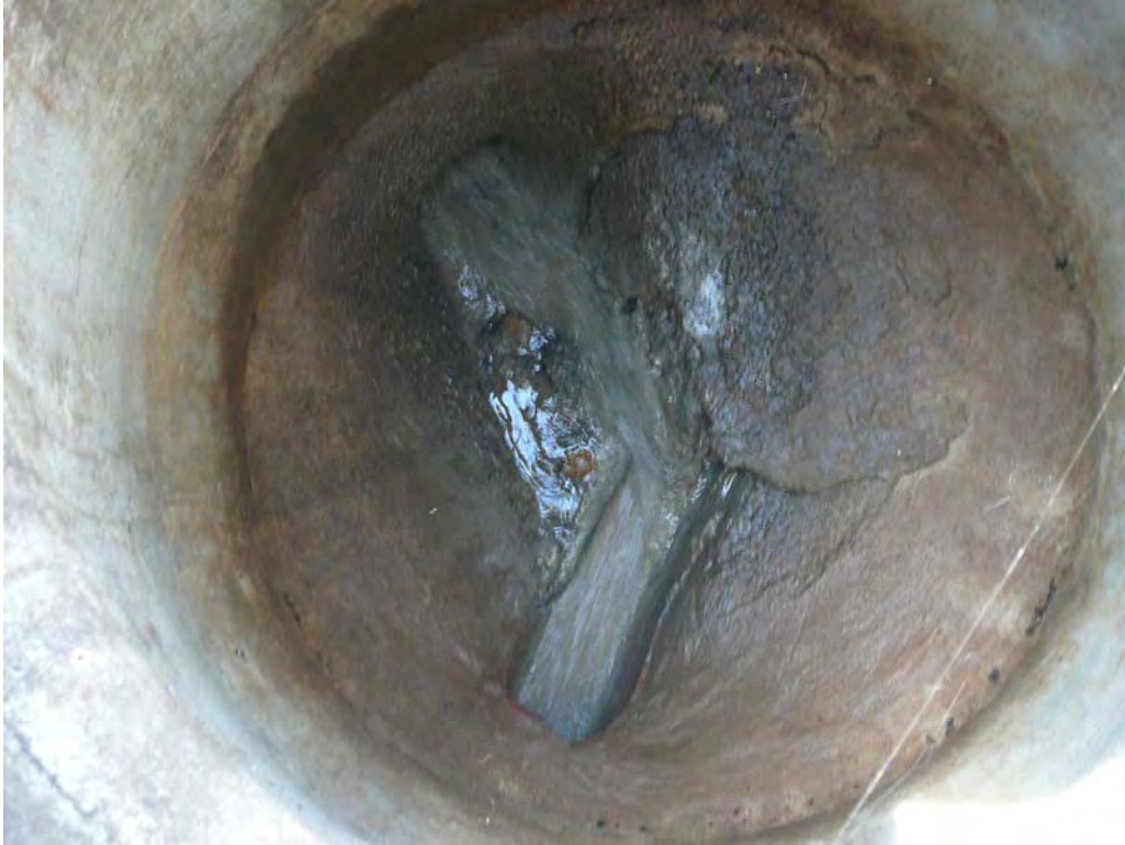
Photo 9 "Ocean View & Coventry" - reduced 90 degree bend in pipe to prevent overflows
