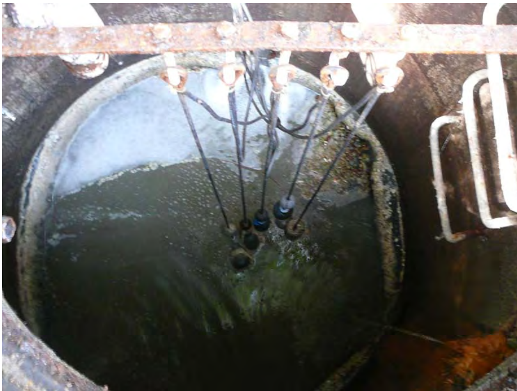
Photo 6 Cannon pump station wet well
