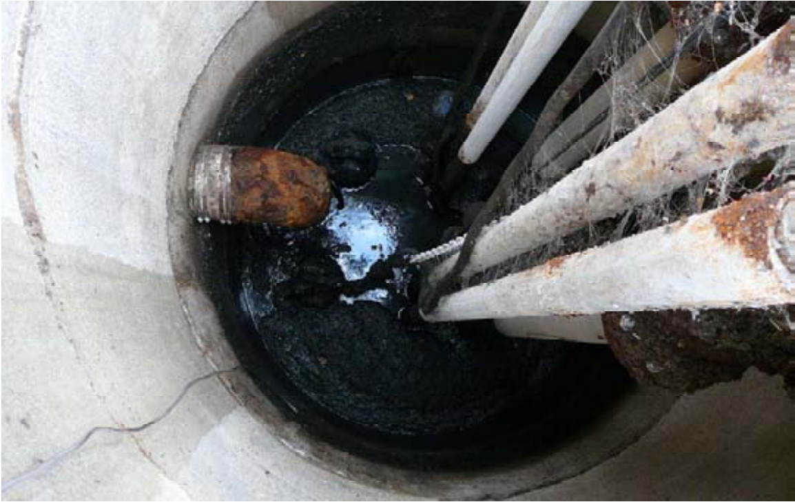
Oakland Photo 9: Denton Place PS wet well.
