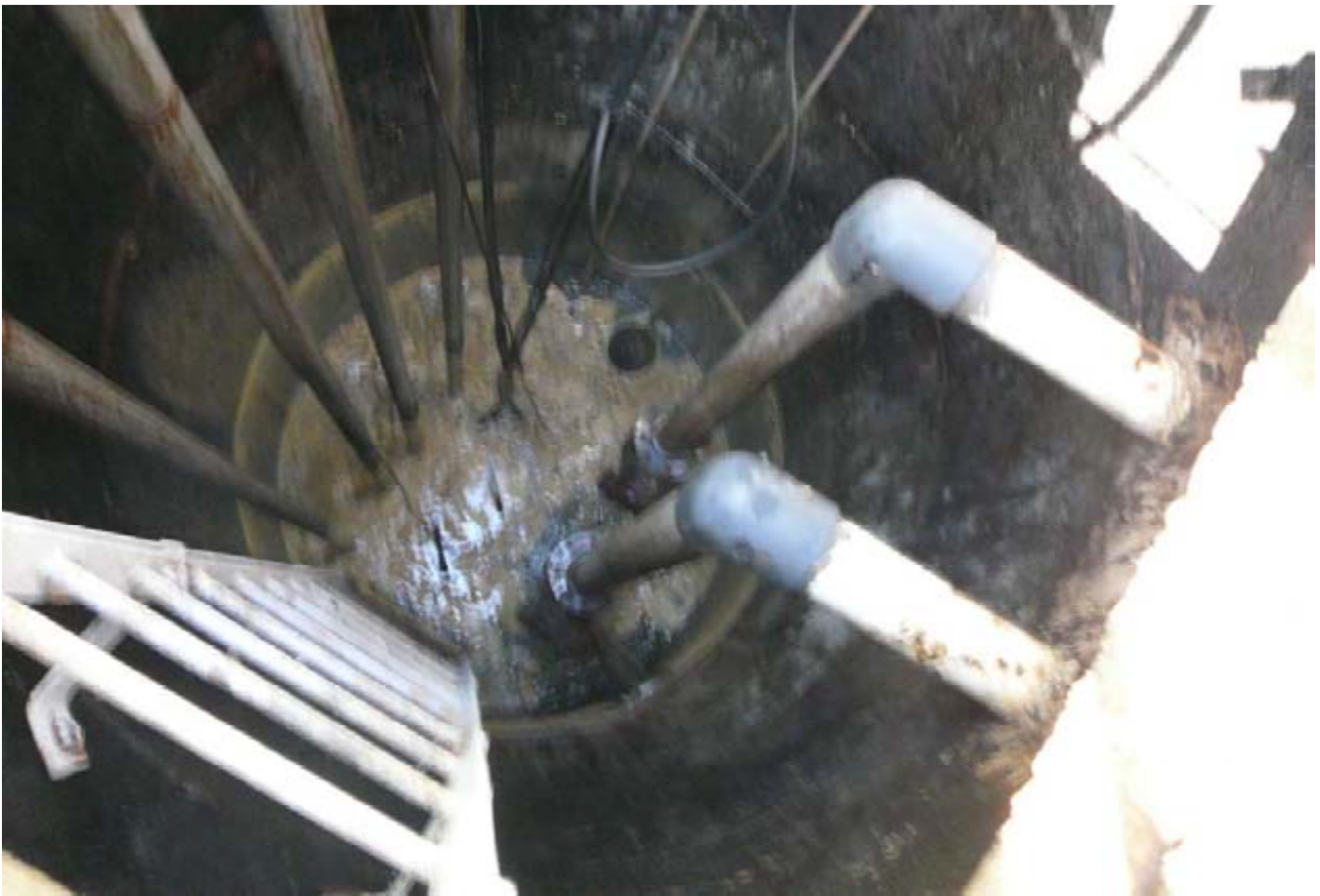
Alameda Photo 3 - Dublin pump station wet well
