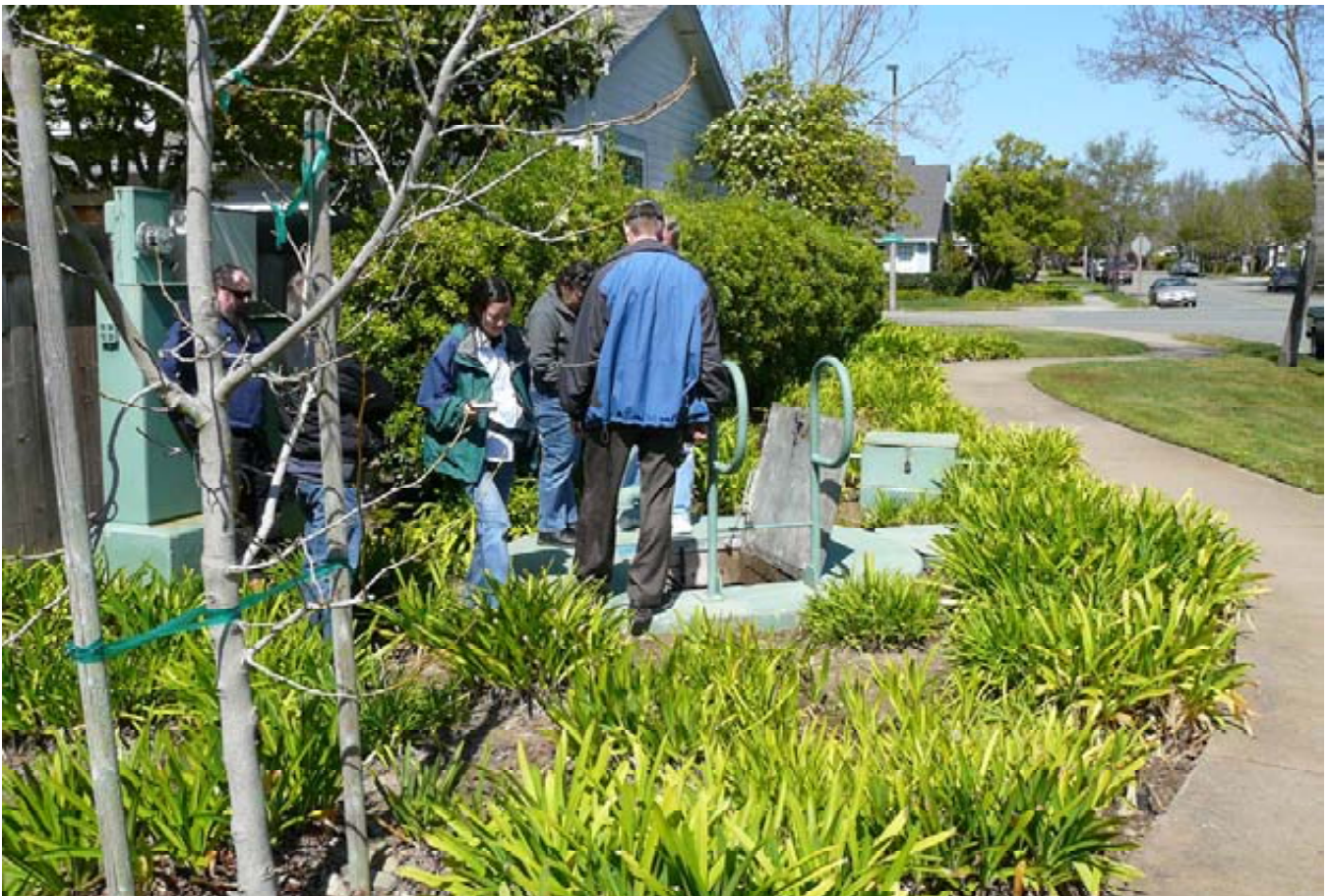
Alameda Photo 4 - Dublin pump station
