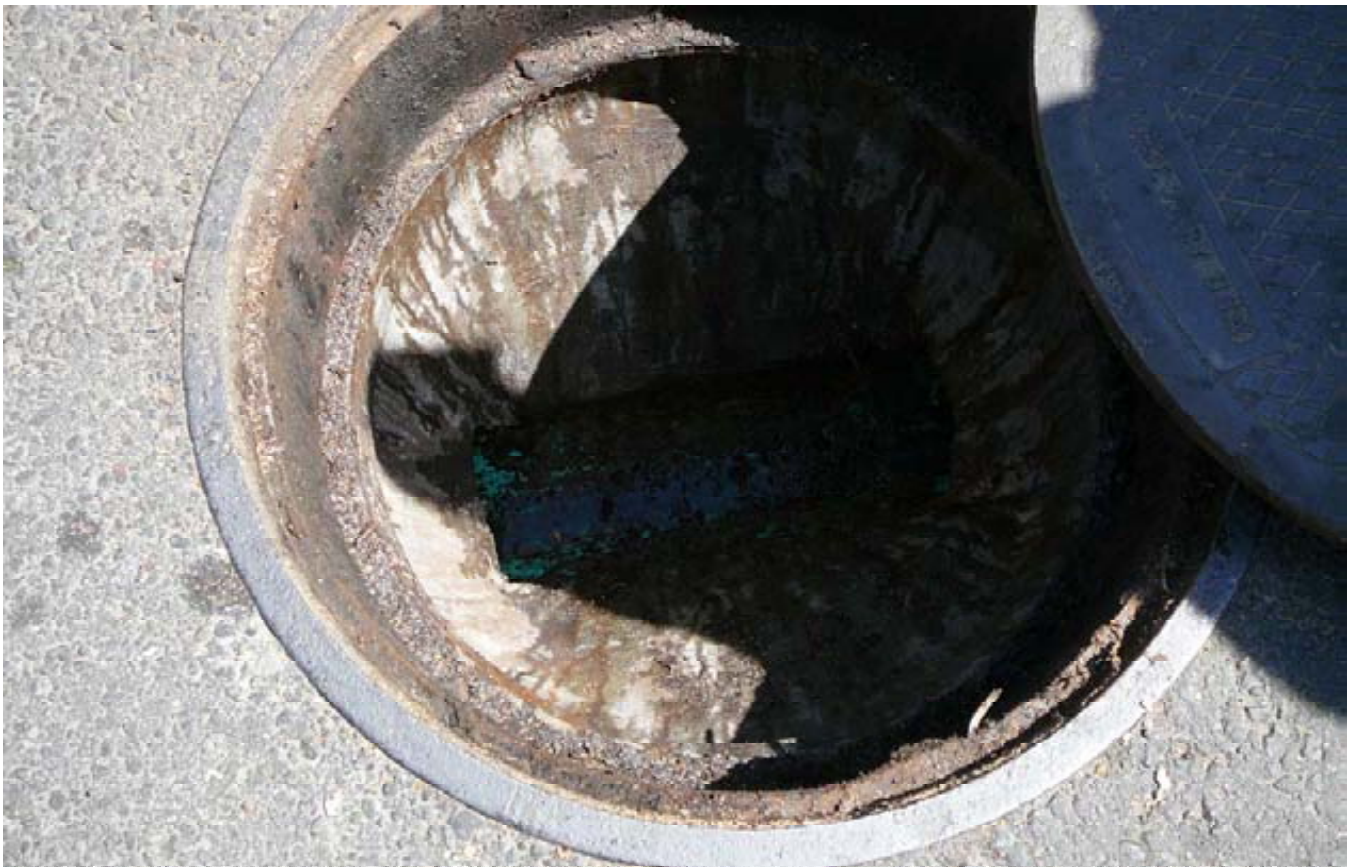
Alameda Photo 9 - Spill site at Alameda Federal Center - Manhole that overflowed
