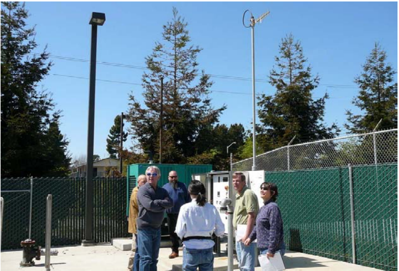
Alameda Photo 11 - Lift station 6
