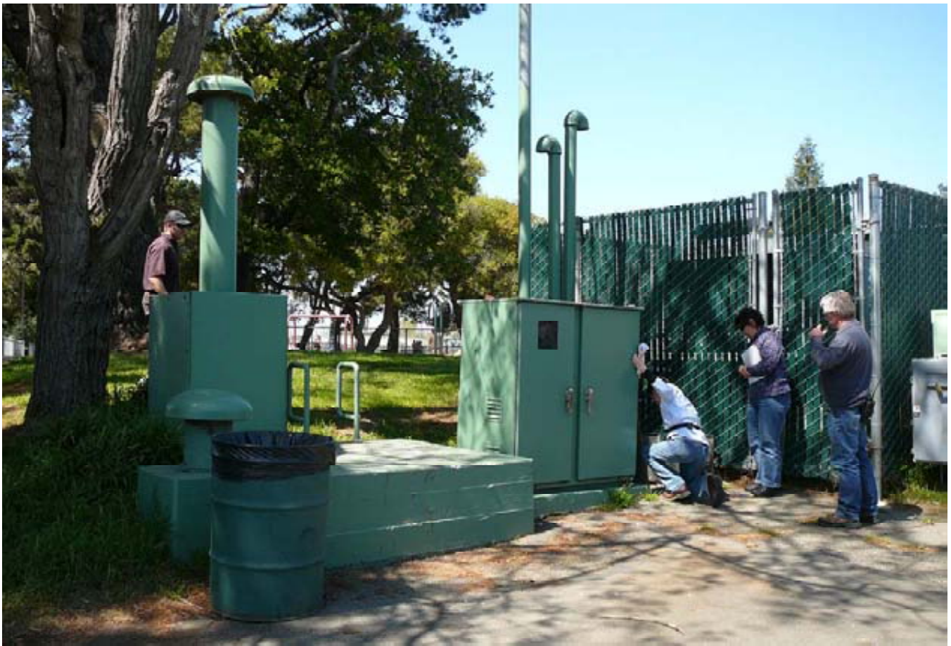
Alameda Photo 7 - 8th and Portola pump station
