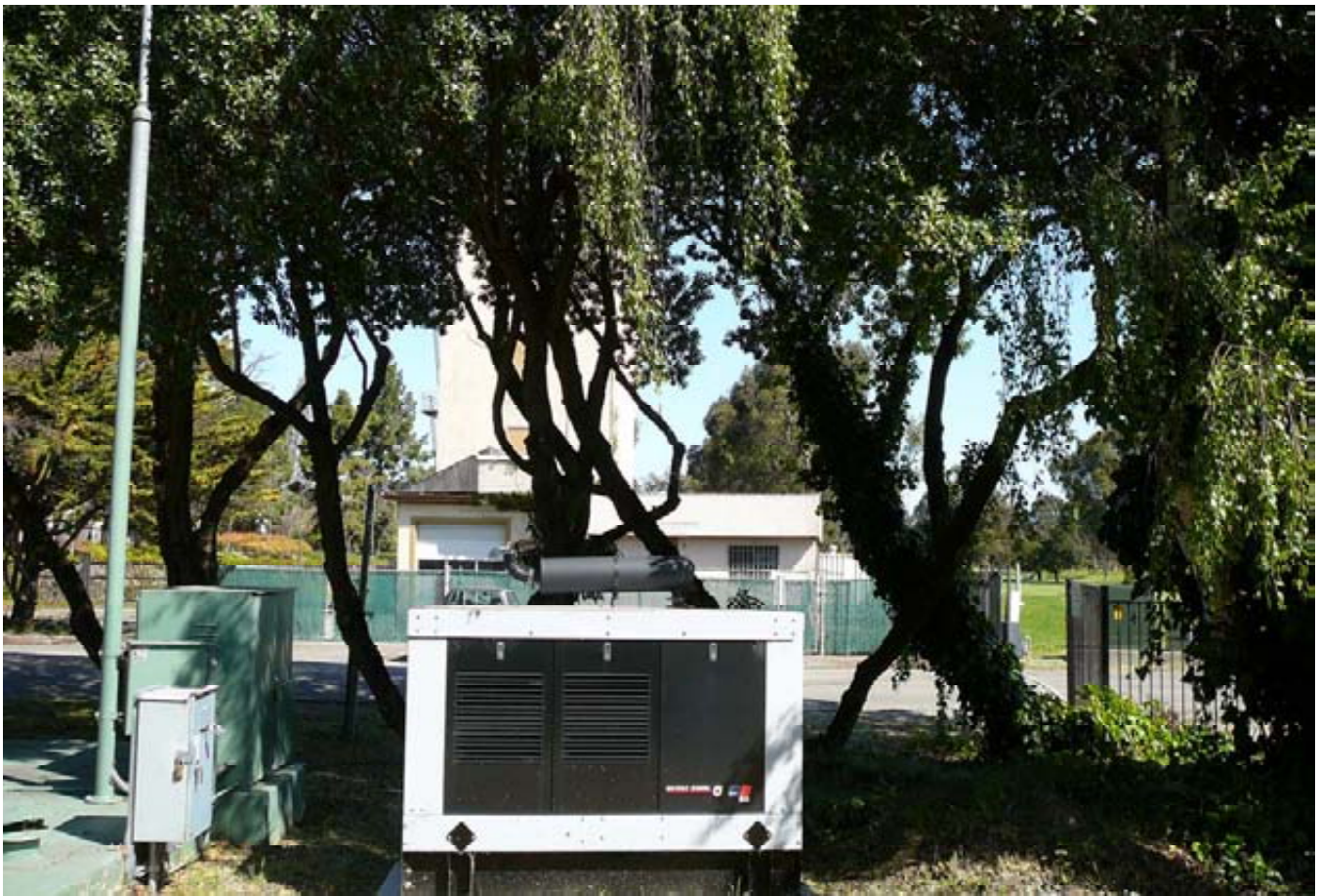
Alameda Photo 1 - BFI pump station
