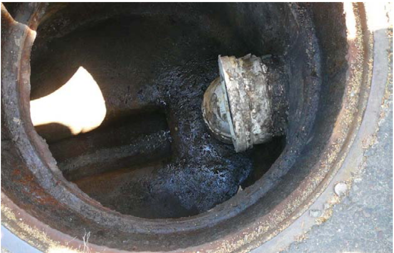
Alameda Photo 10 - Spill site at Alameda Federal Center - Second manhole showing pipe fix
