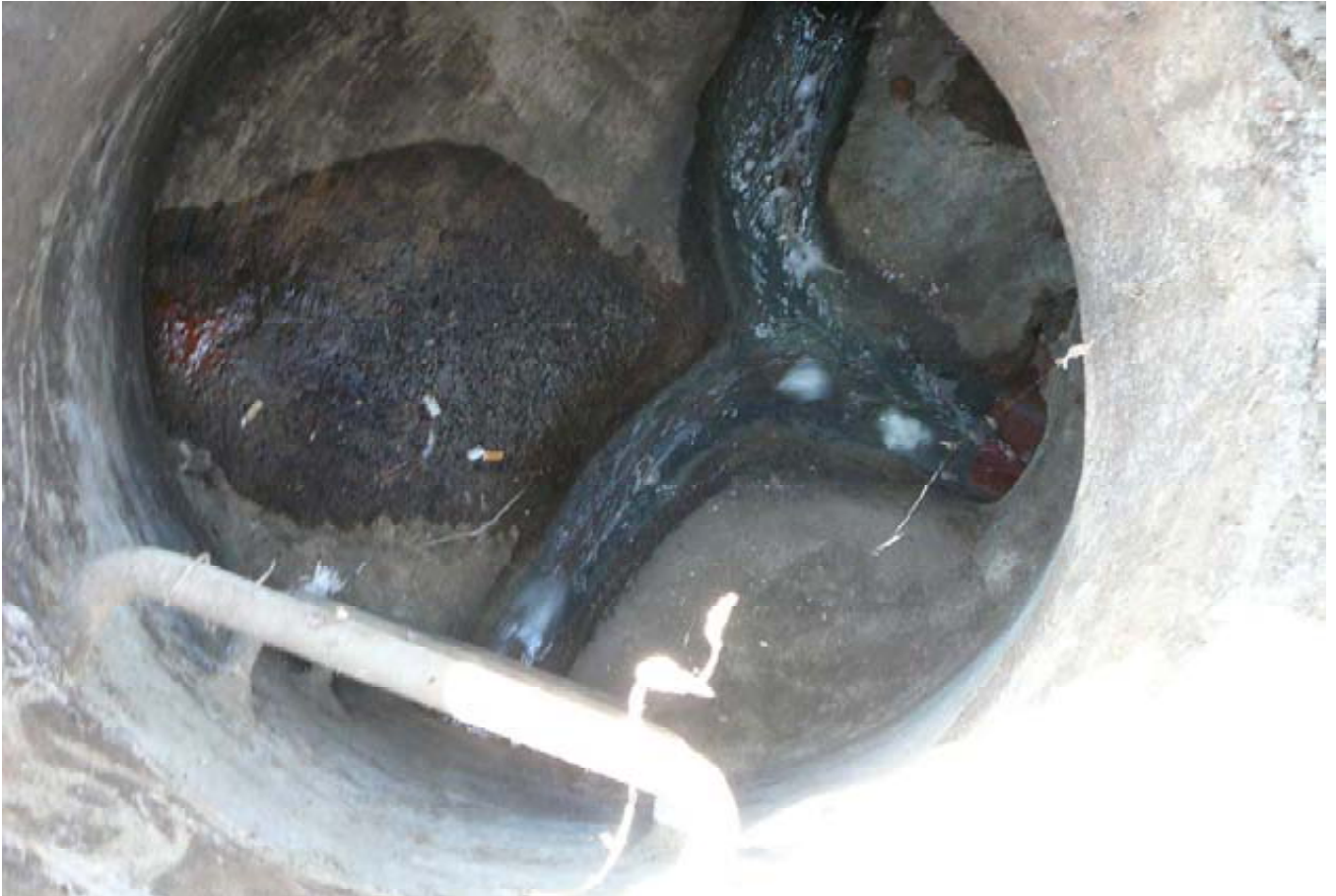
Alameda Photo 16 - Kitty Hawk spill site manhole
