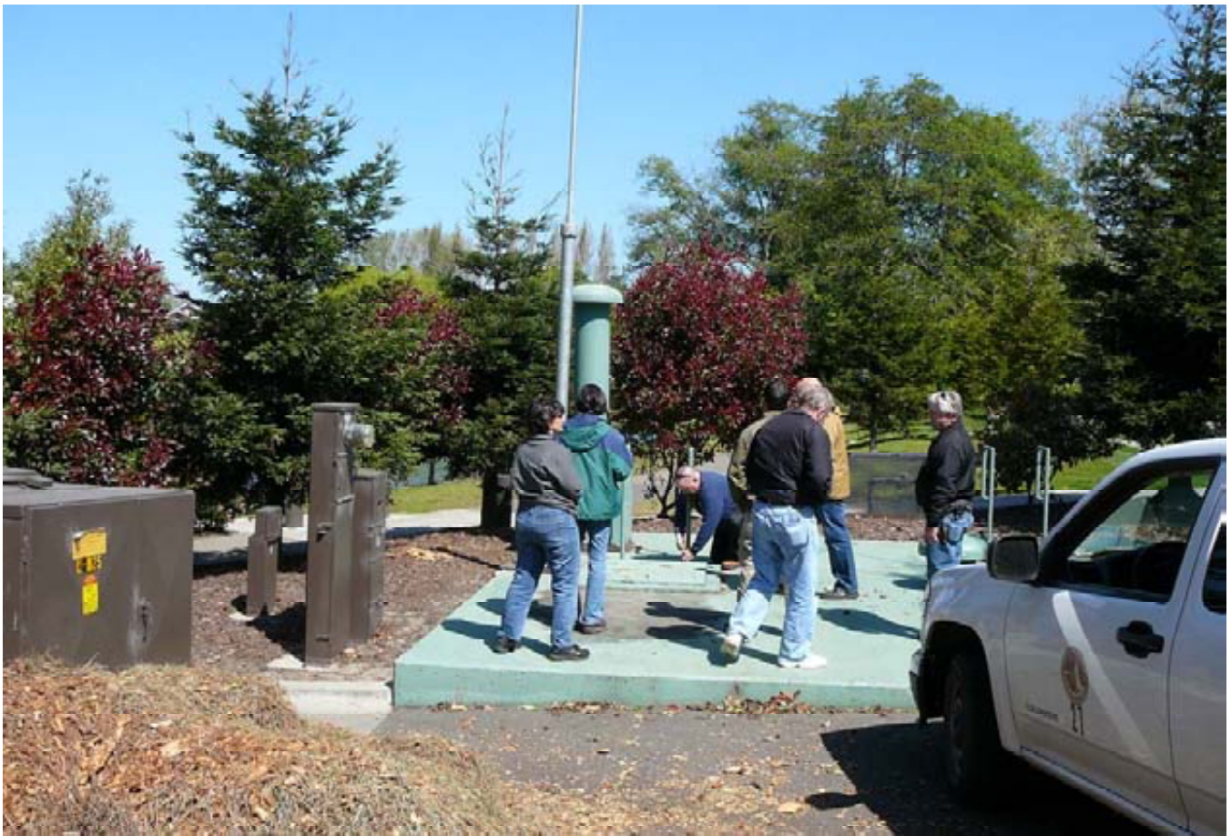
Alameda Photo 5 - Catalina pump station
