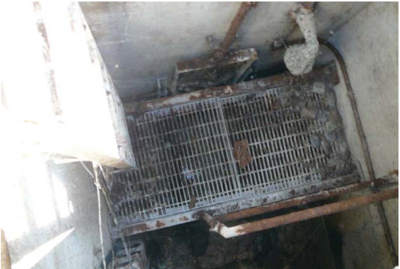
Alameda Photo 6 - Catalina pump station wet well
