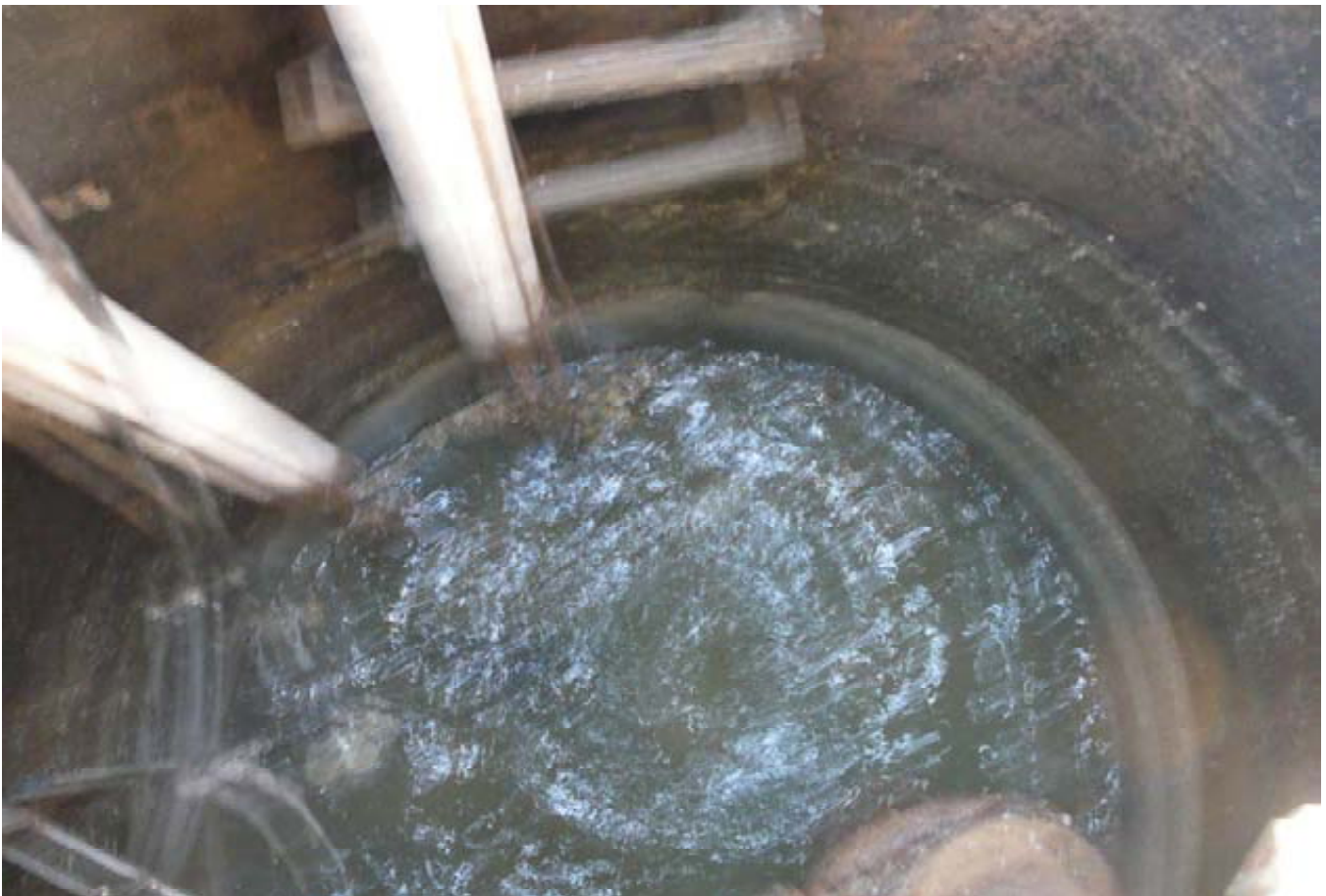
Alameda Photo 14 - Willow pump station wet well
