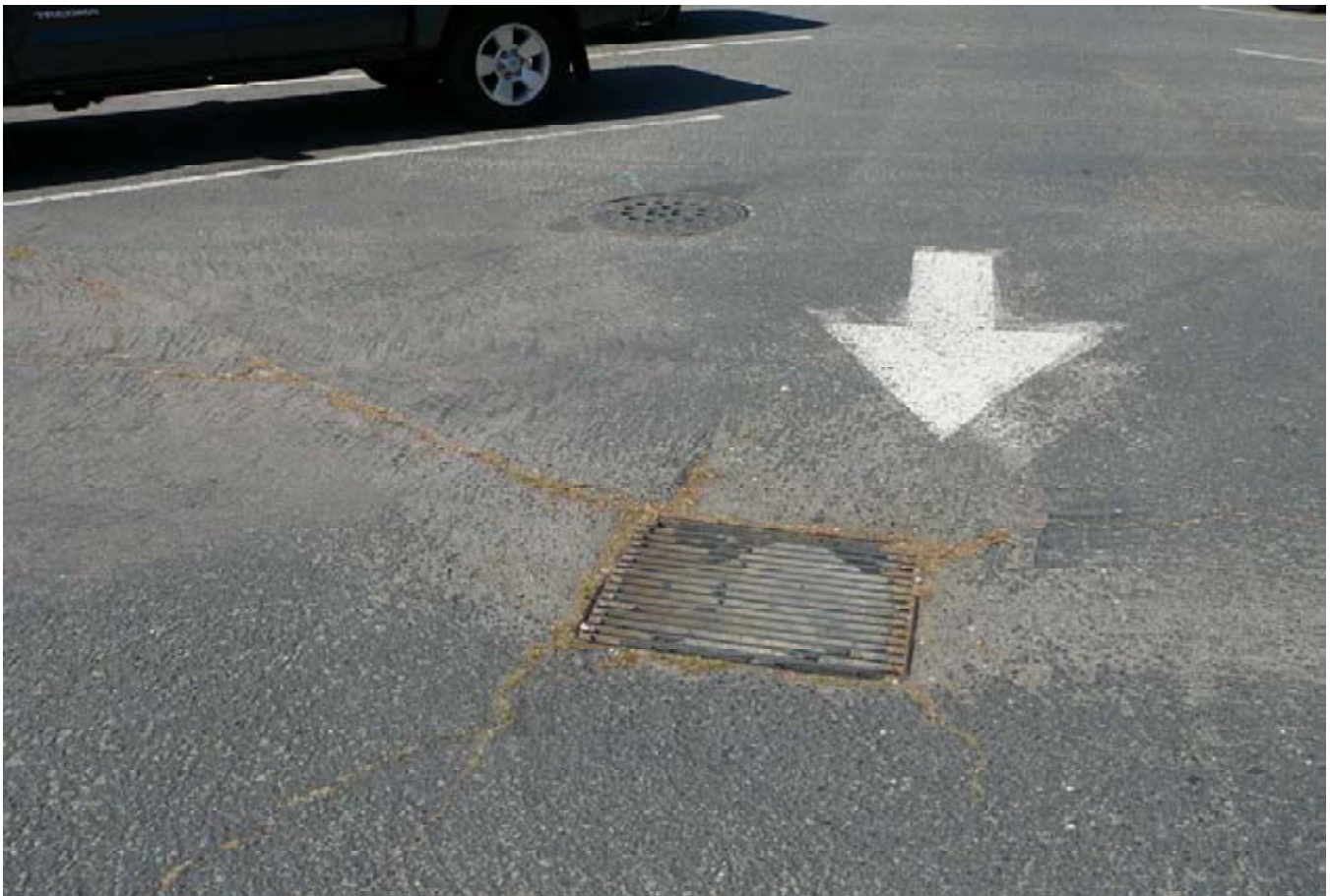
Alameda Photo 2 - Location of overflow from BFI pump station
