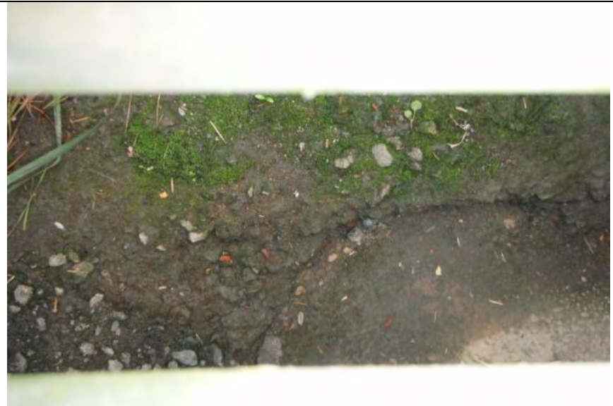
Photograph 2 – View into storm drain inlet pictured in Photograph 1 (Note: Sediment accumulation within inlet)
