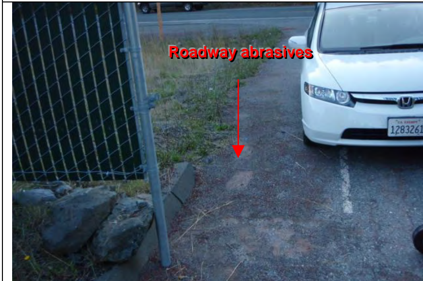
Photograph 7— Roadway abrasives outside facility entrance
