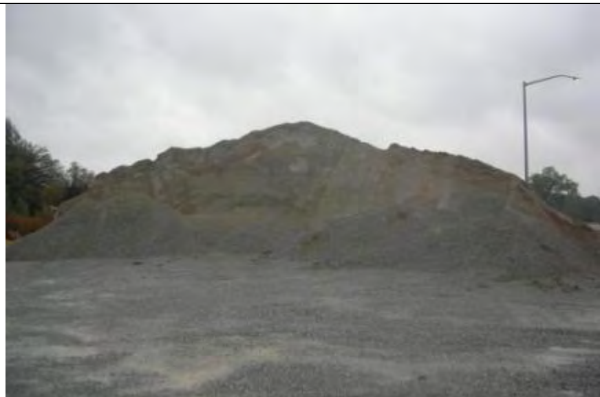
Photograph 2 – Lack of BMPs to contain stockpiled materials
