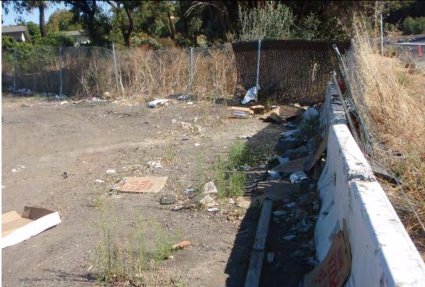
Photograph 5 – Example of fugitive trash and debris
