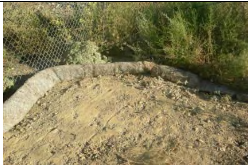
Photograph 3 – Close up view of straw wattle installation shown in Photograph 2
