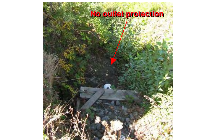
Photograph 11— Outlet pipe down-gradient of facility outfall
