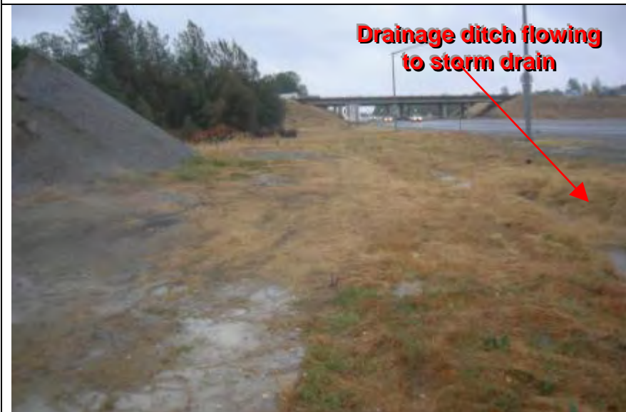
Photograph 3 – View of Photograph 2 stockpile proximity to drainage ditch
