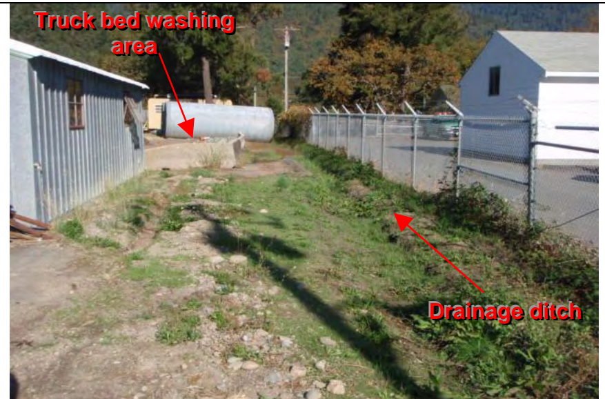
Photograph 14 – View of drainage ditch along southern edge of facility
