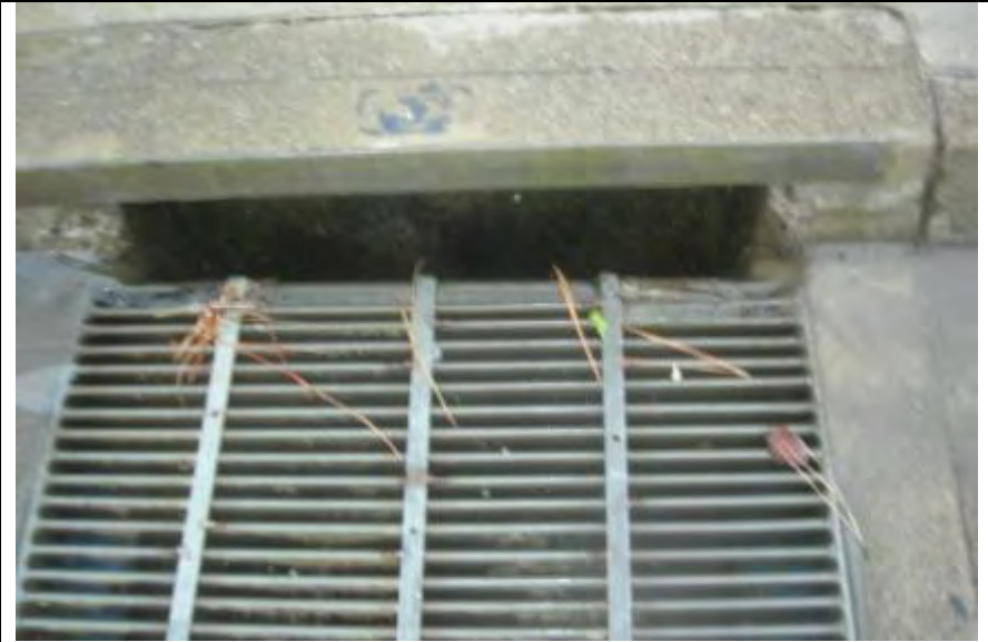
Photograph 2 – Storm drain from Photograph 1
