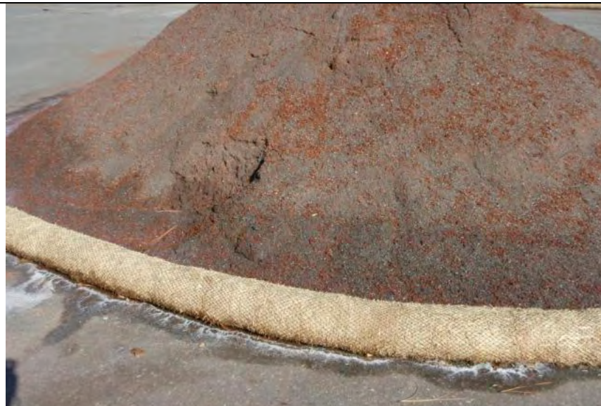
Photograph 7— Closer view of straw wattle BMP around stockpile (Note: Apparent salt residue)
