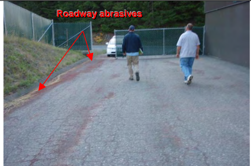
Photograph 6 – Roadway abrasives on impervious ground surface
