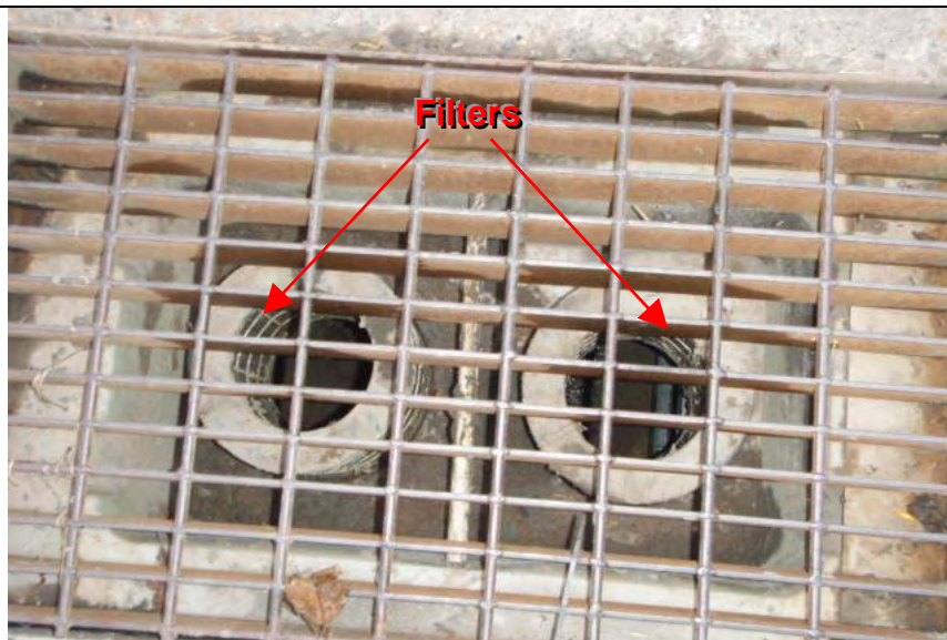
Photograph 8 – View into another storm drain inlet at the facility
