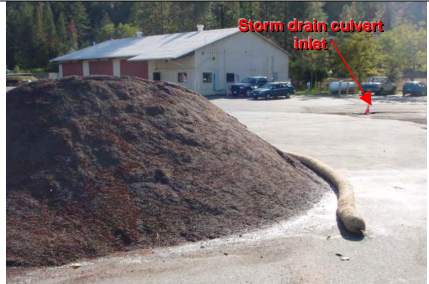
Photograph 6 – Inappropriate application of straw wattle BMP
