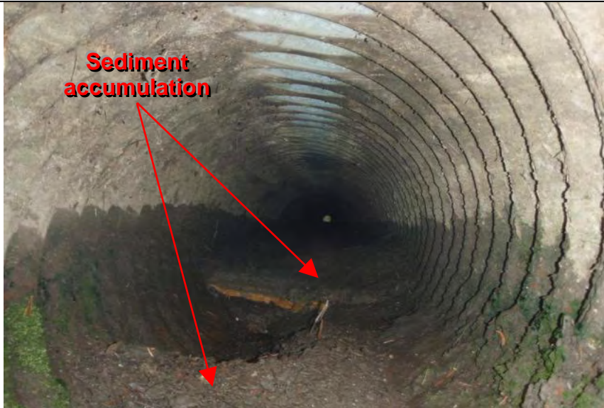
Photograph 5— View into storm drain pipe from outlet
