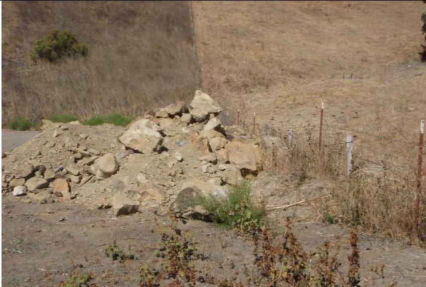
Photograph 5 – Note lack of BMPs for containment around stockpile and the stockpile's proximity to the fenceline
