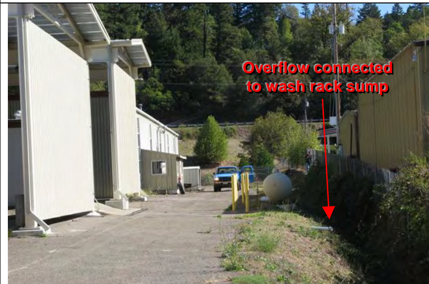
Photograph 3 – Sump overflow leading to drainage ditch
