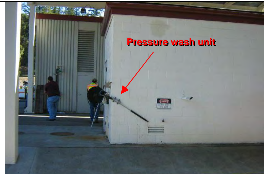
Photograph 1 – Covered wash rack
