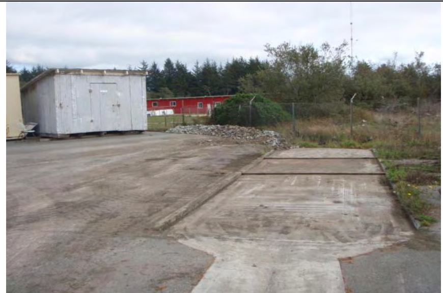
Photograph 6 – Area used for stockpiling washout material (Note: Sediment accumulation on impervious ground surface)
