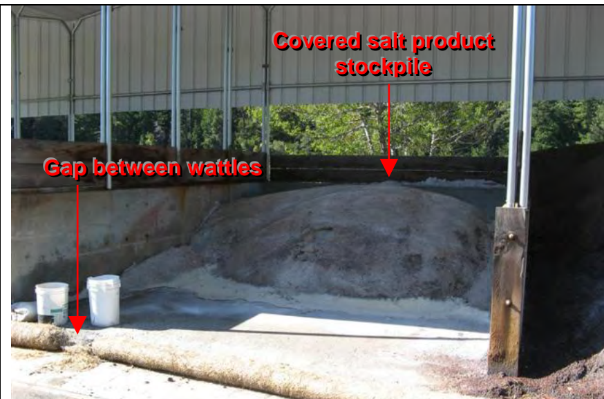
Photograph 9— Inappropriate application of wattles
