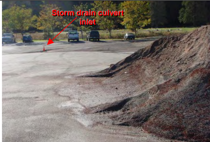
Photograph 5— Stockpile of sand and ash mixture up-gradient of inlet
