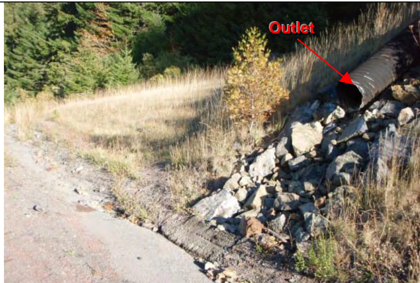
Photograph 3 – Discharge location from inlet shown in Photograph 2
