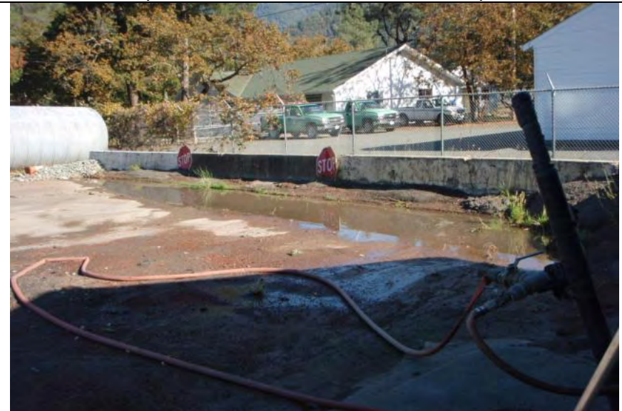
Photograph 12 – Bermed area used for truck bed washing
