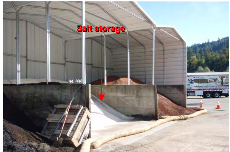
Photograph 8 – Inappropriate application of straw wattle BMP
