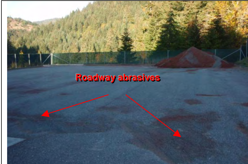
Photograph 5— Roadway abrasives on impervious ground surface
