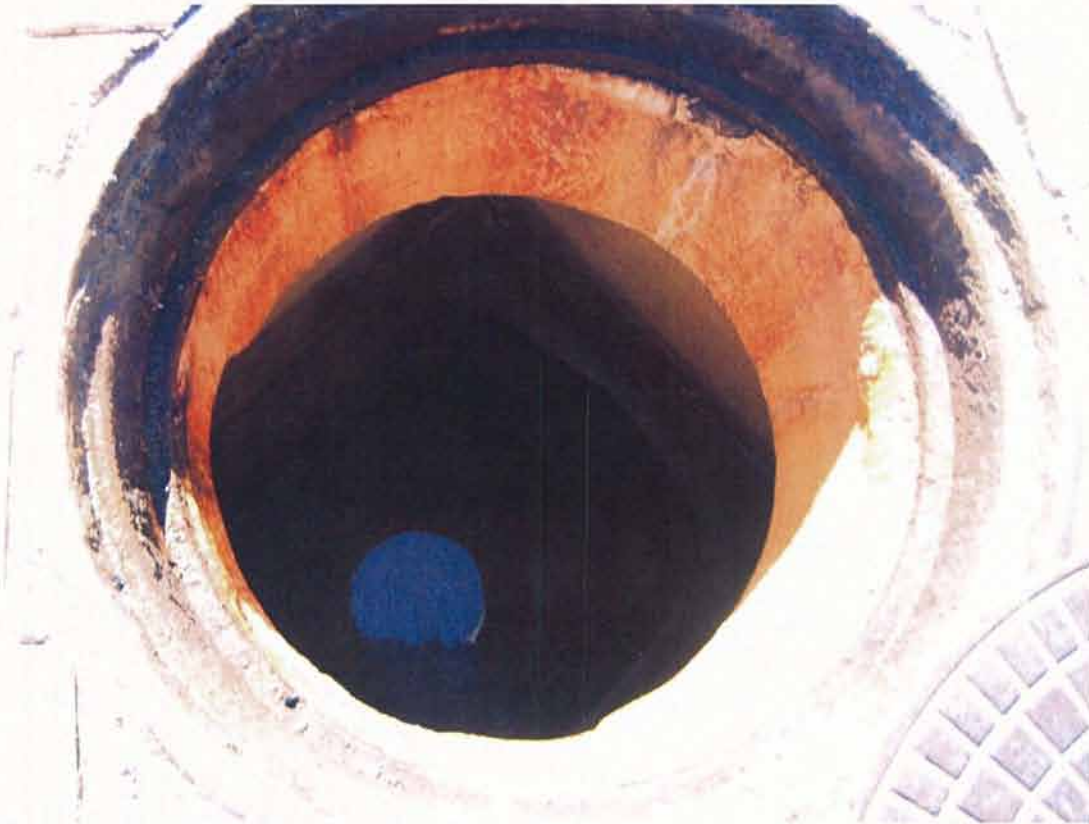
Figure 2: IMG_3260. Low-flow diversion system.
