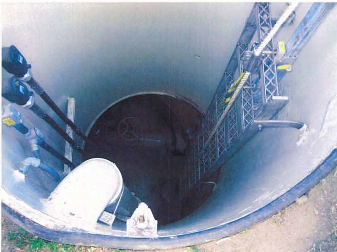
Figure 5: IMG_3263. Catherine lift station.
