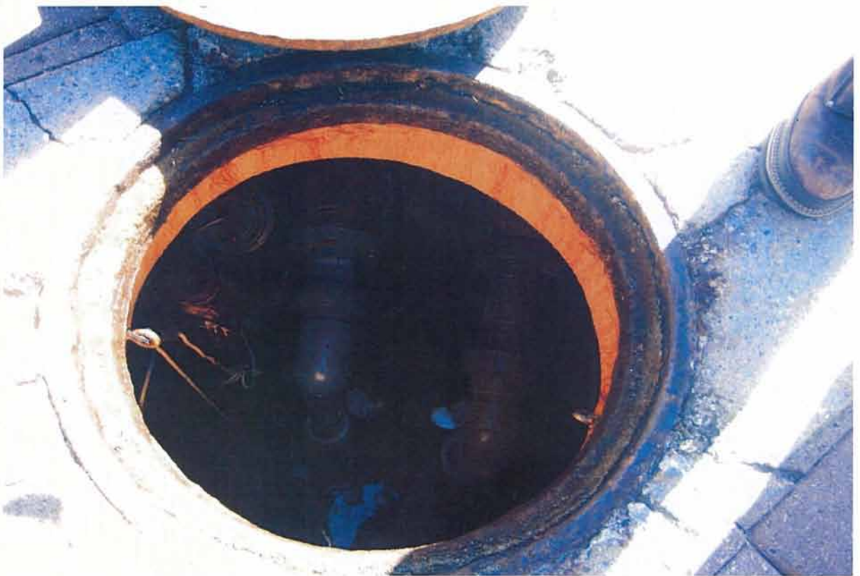
Figure 1: IMG_3259. Pump station for the low-flow diversion station at “Busy Bee” location. The City told the inspection team that the sewer system uses the low-flow diversion system to capture sewer system spills, which can then be pumped back to the WWTP. The system is a separate sewer system but is, in effect, operated similarly to a combined system.
