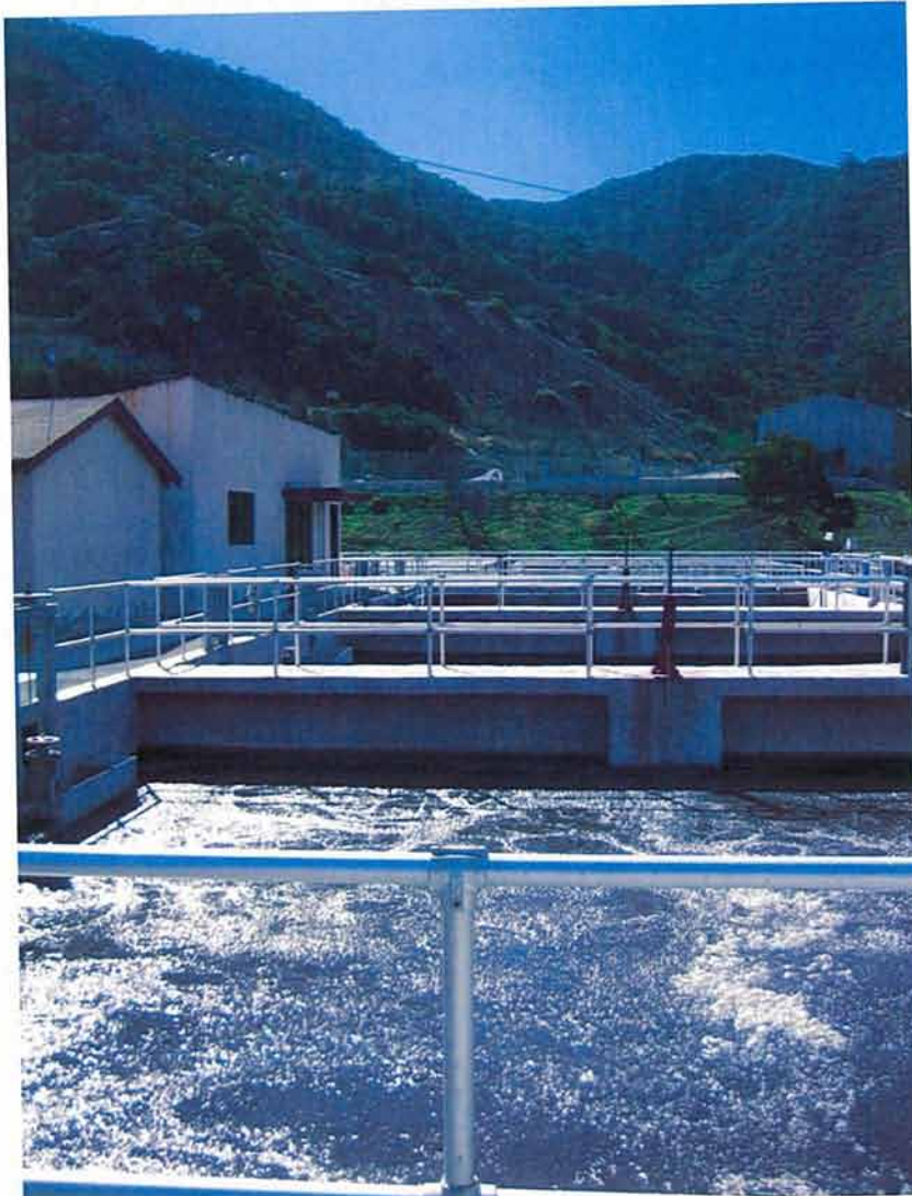
Figure 14: IMG_3272. Aeration basins. Original image has been rotated 90° clockwise.
