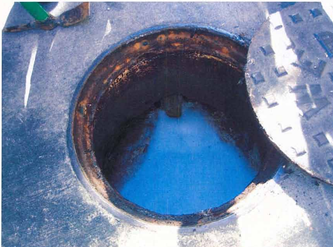
Figure 3: IMG_3261. Manhole located in the alley behind the El Galleon restaurant. Small amount of grease is visible, lots of soap suds.
