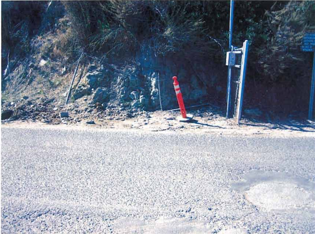
Figure 6: IMG_3264. Low point manhole between Catherine & Pebbly Beach lift stations.
