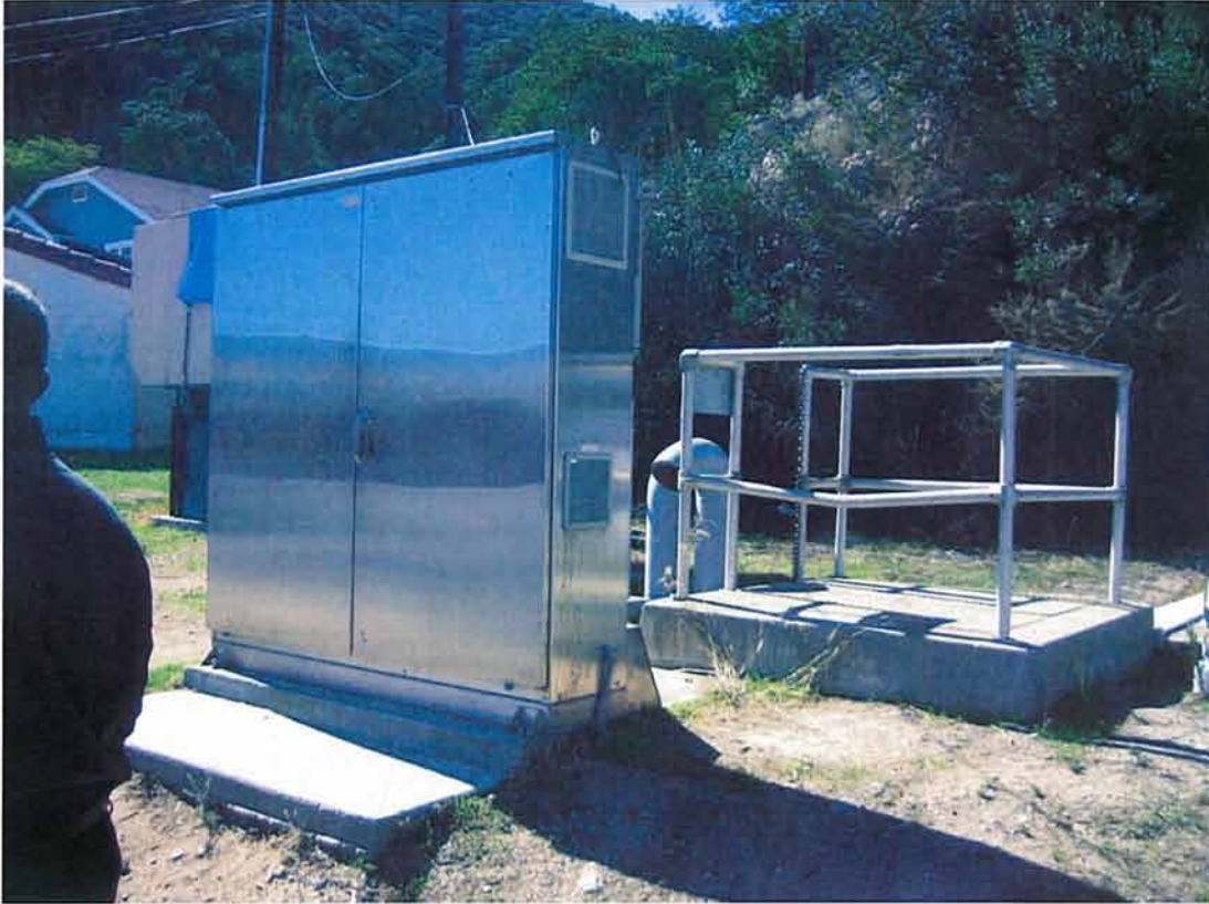
Figure 10: IMG_3268. Control panel and wet well area at Pebbly Beach lift station.
