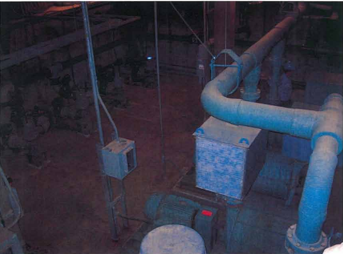
Figure 17: IMG_3275. Pumps and blowers.
