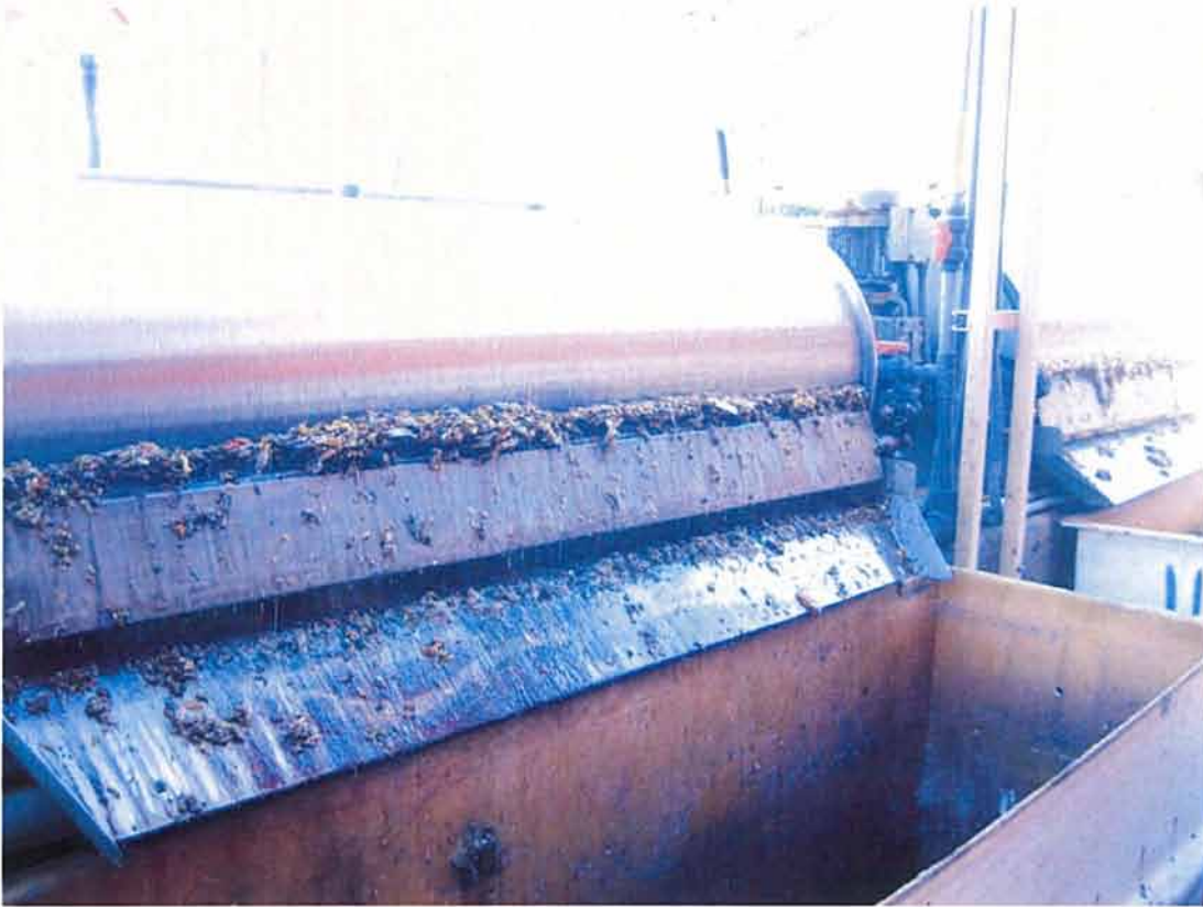
Figure 11: IMG_3269. Rotoscreens at wastewater treatment plant, site of an in-plant spill.
