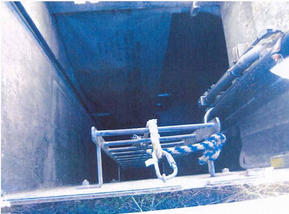
Figure 9: IMG_3267. Pebbly Beach lift station.
