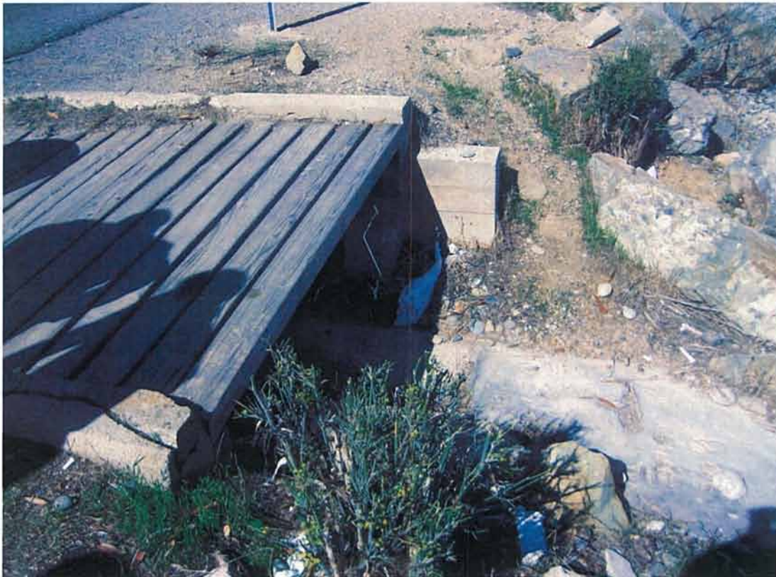
Figure 7: IMG_3265. Outlet to beach from the low point manhole pictured in IMG_3264.
