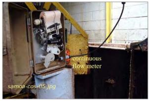
Photo #8: NPDES Sample Point - Flow Meter
