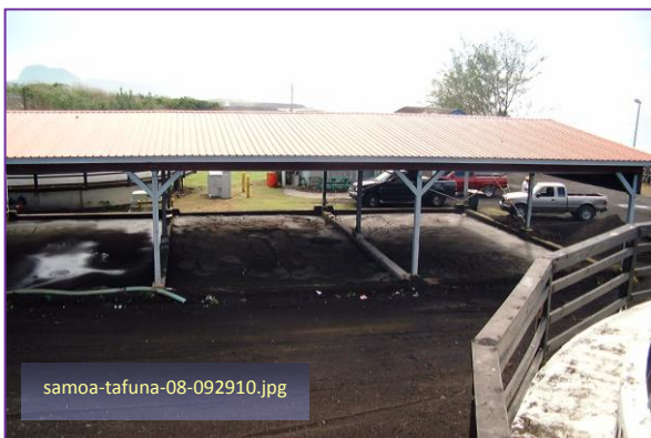
Photo #5: Tafuna STP – Sludge Drying Beds No.1 Taken By: Greg V. Arthur Date: 09/29/10
