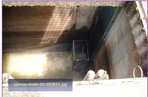
Photo #8: Utulei STP – Wet-Well and Cage Barscreen Taken By: Greg V. Arthur Date: 09/28/10
