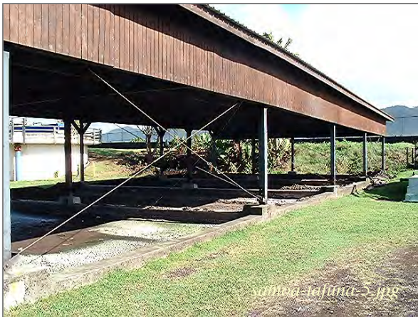
Photo: Tafuna STP – Sludge Drying Beds Taken By: Greg V. Arthur Date: 07/16/07
