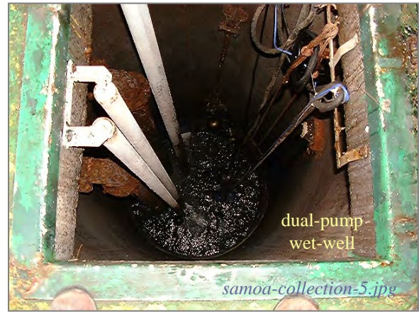
Photo: ASPA Sewers – Fagaalu Lift Station Taken By: Greg V. Arthur Date: 07/17/07
