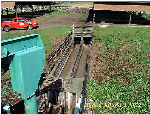
Photo: Tafuna STP – Headworks Taken By: Greg V. Arthur Date: 07/16/07
