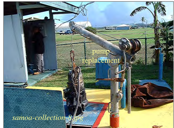
Photo: ASPA Sewers – Airport Lift Station Taken By: Greg V. Arthur Date: 07/17/07
