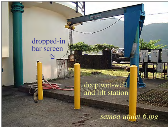
Photo: Utulei STP – Inlet Lift Station Taken By: Greg V. Arthur Date: 07/16/07
