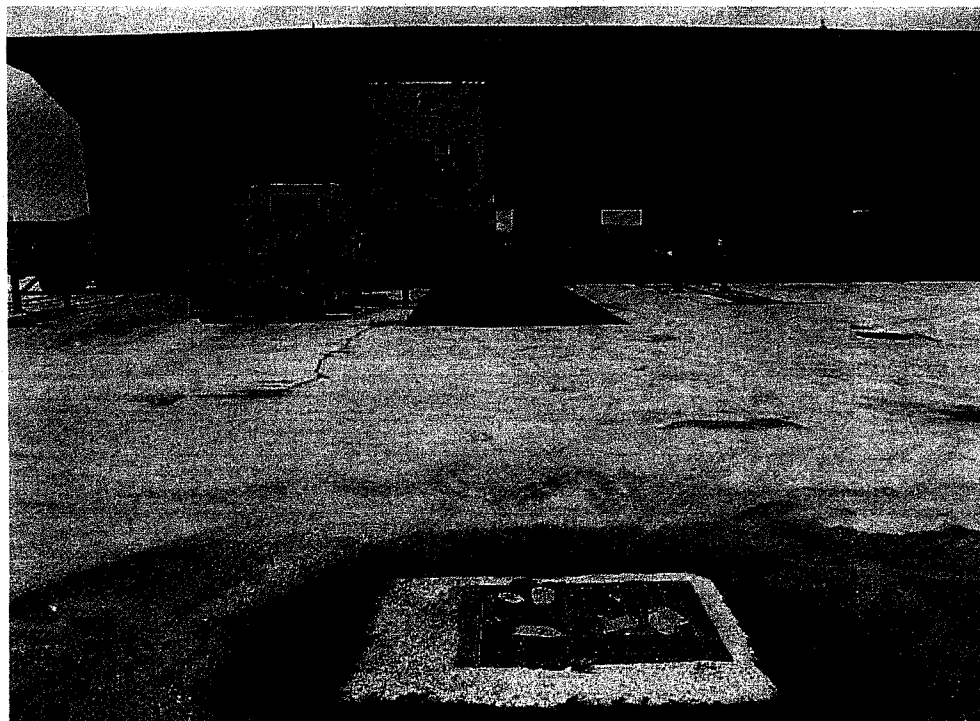
Photo 6 - Close-up of storm drain inlet outside of Matson's maintenance area
