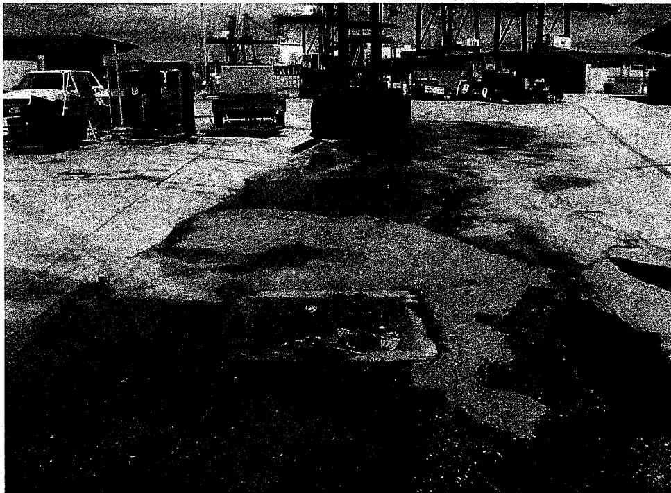
Photo 2 - Drain inlet closeby the Port Authority's equipment and repair building
