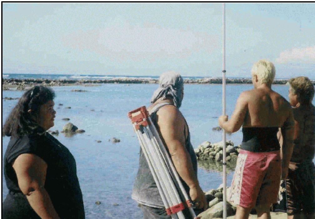
Figure 102, Ancient Fishpond, Modern Tools. Rebuilding Kahinapohaku Fishpond.
