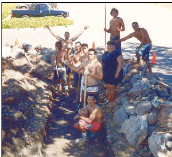
Figure 2. Trainees Building Dry Stack Stone Wall at Kulana O'iwi.
