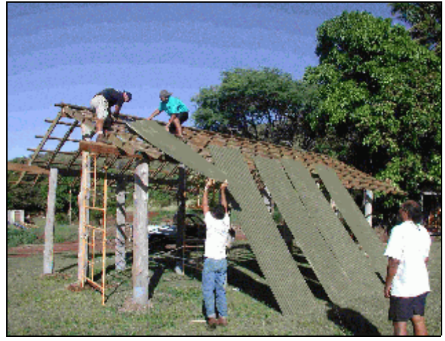
Figure 52, Constructing the Hale at Keawanui.
