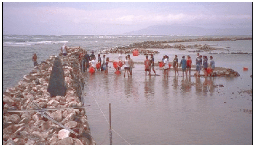
Figure 4. Kahinapohaku Fishpond. Passing 'ili'ili , small stones, to the fishpond wall using red plastic baskets.
