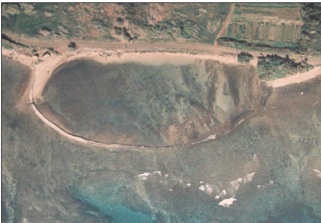
Figure 35, Kahinapohaku Fishpond About Midway Through Wall Restoration.
