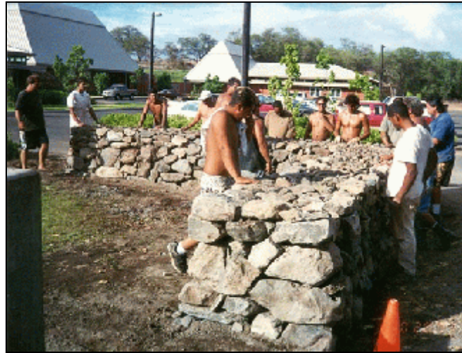
Fig. 80, 81; Hands-on Dry Stack Rock Wall Building Class at Kulala O'Iwi.
