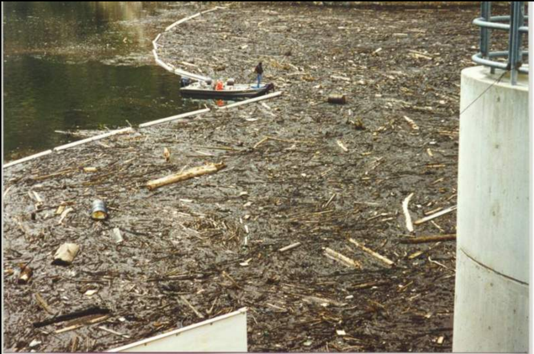
Strontia Springs Reservoir after 1996 Buffalo Creek Fire
