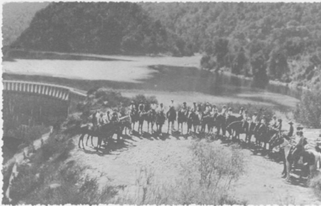
San Clemente Dam • March 29, 1932
