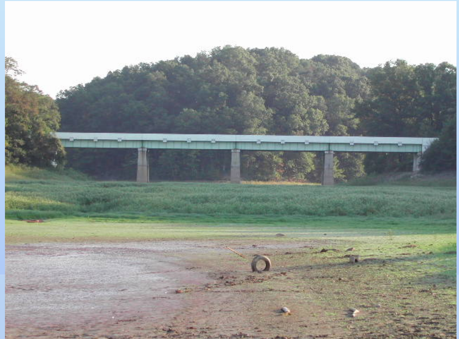
Prettyboy Reservoir, Maryland during 2002 drought. Photo courtesy of National Weather Service.
