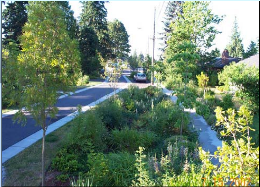
↑ Street right-of-way bioswale
