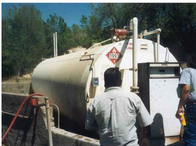
Upper left: Good example of secondary containment.
