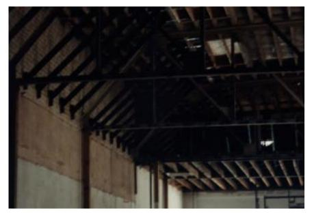
Almost two tons of drywall were collected in 4 yard roll-off containers and hauled to Ventura County to be used as soil amendment. Hundreds of board feet of wood framing members were salvaged, including old growth dimensional lumber in 2 x 4, 2 x 6, and 2 x 8 sizes. These were denailed and set aside for reuse on this and other projects. Only two small dumpsters (1 ton total weight) were taken to the landfill.
