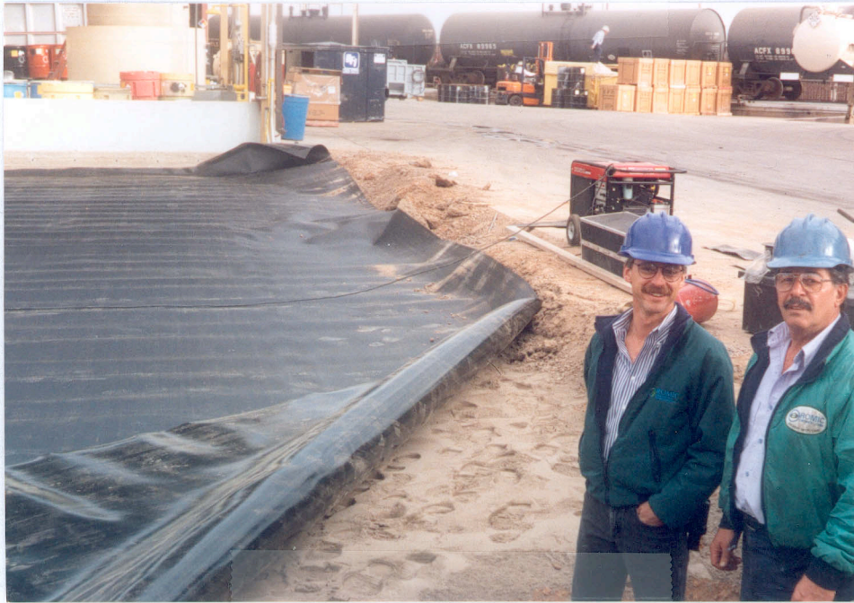
Liner being unrolled under tank farm
