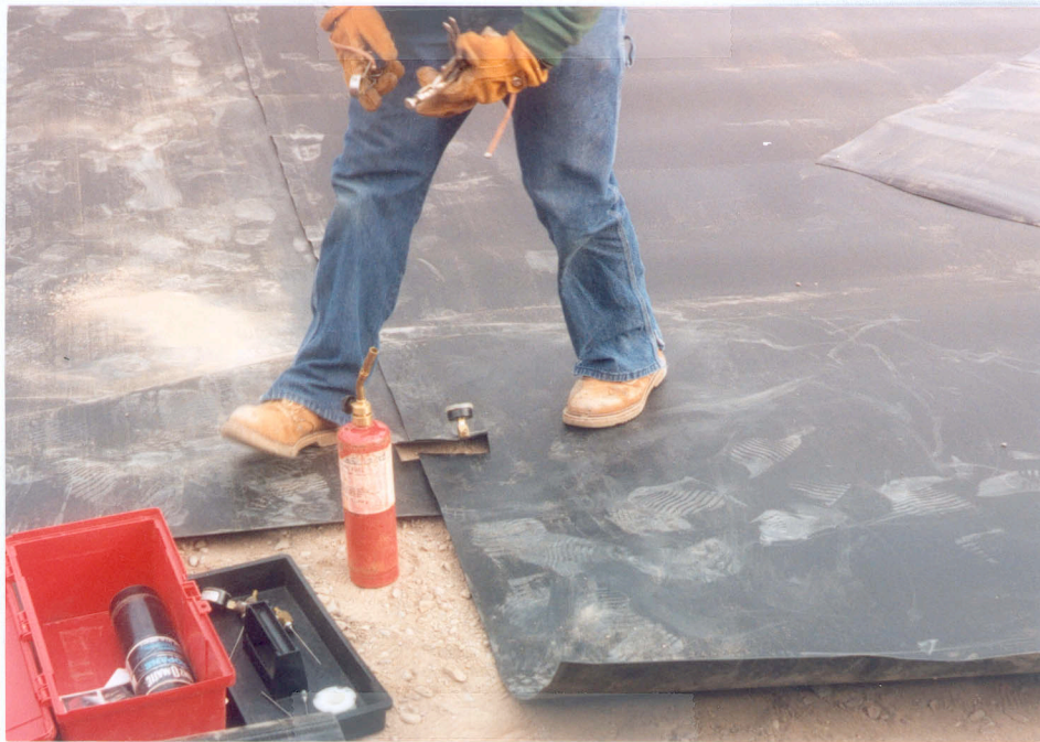
Liner seal being tested for leaks
