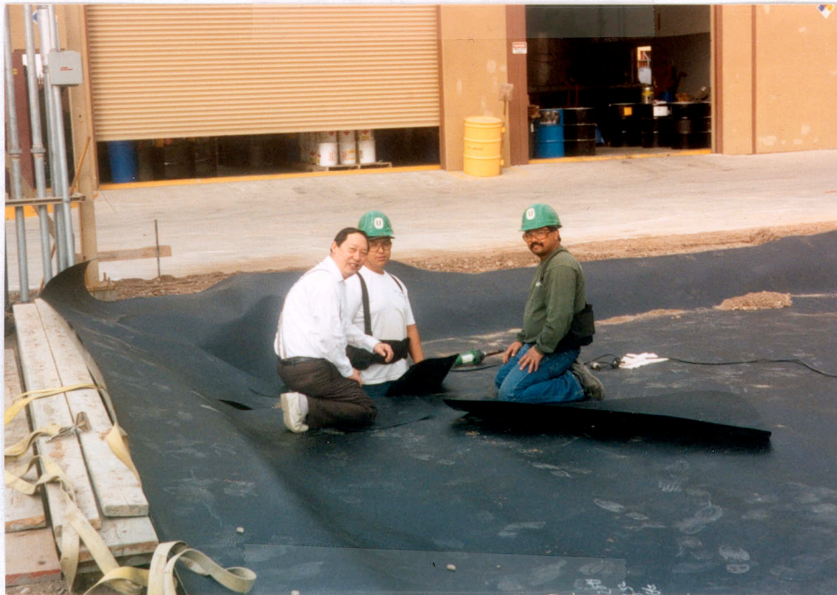
Sump area for liner being installed
