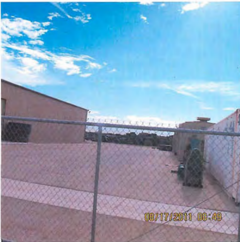
View from the southwest corner of the former Specialty Alloys site. Note the large tires adjacent to the building. All the photos in the current survey of the former Specialty Alloys site are very similar to these. The two large tires have not been moved.
