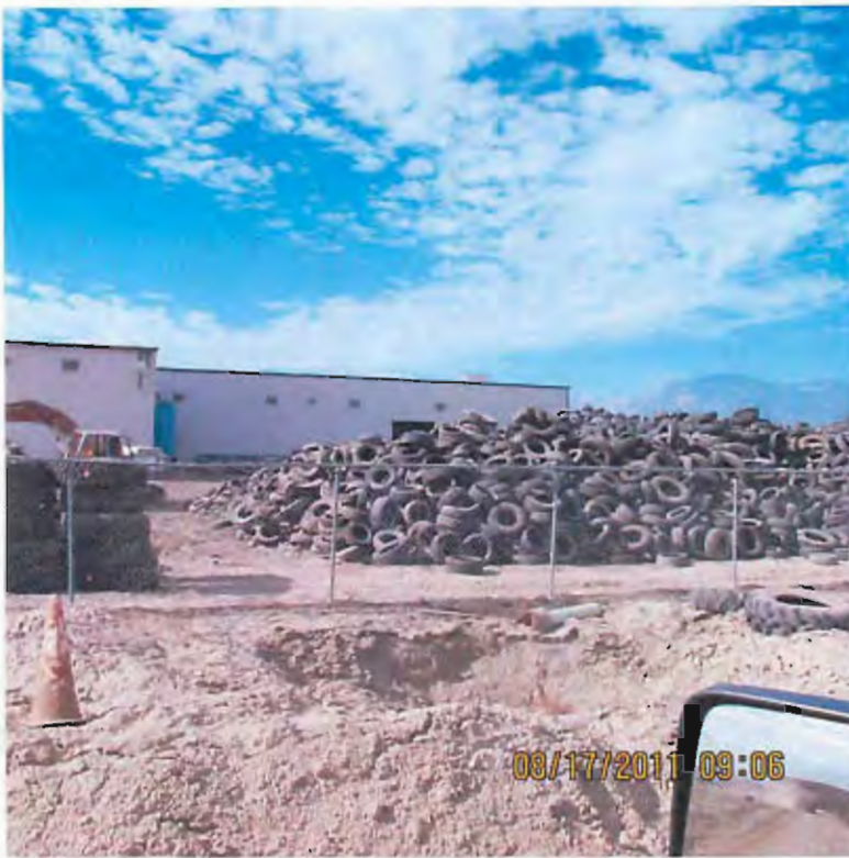
A view of the aisle with the tire handling equipment from outside the facility. The current survey photo is very similar. The tires outside of the fence, visible on the right, were placed to form a barrier for a hole that was excavated to repair piping.
