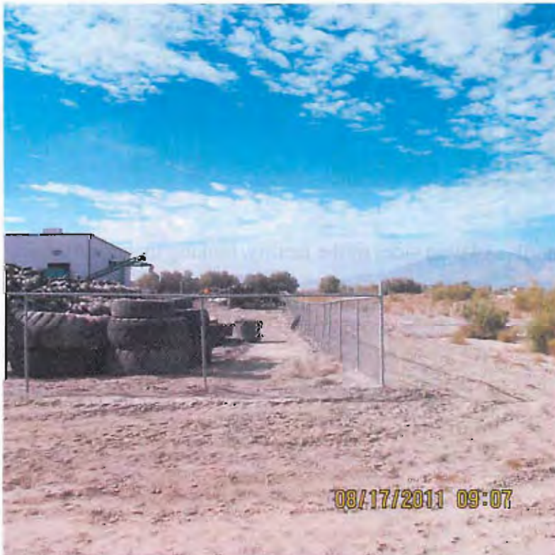
North-west corner of the facility, showing the western fence line. The current survey shows improvement along the west fence line.
