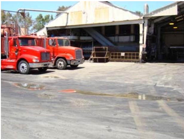
Pumping grease at Salinas Tallow
