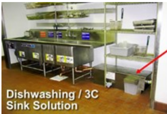
Figure 3. Active Grease Separation units can be installed right after a sink and remove grease and solids from effluent.
