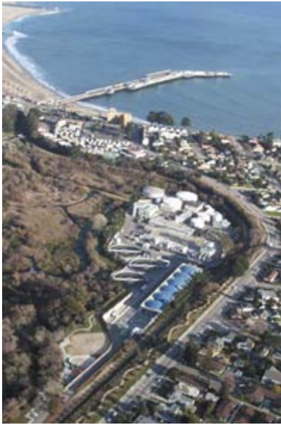
Figure 8. Aerial view of the City of Santa Cruz Wastewater Treatment Facility and the Neary Lagoon .
