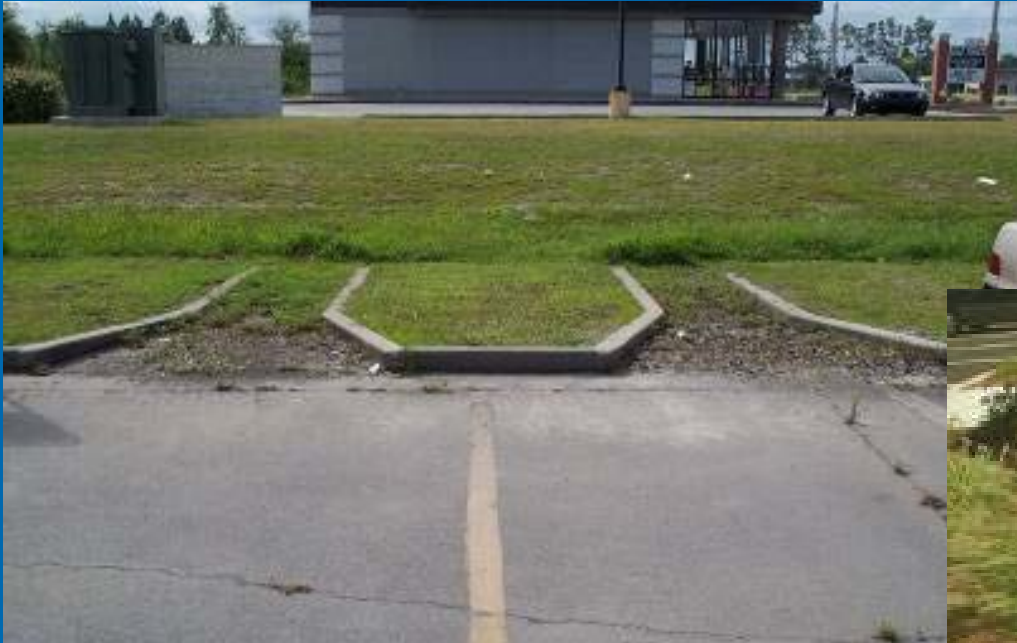
Parking lot drains to swale
