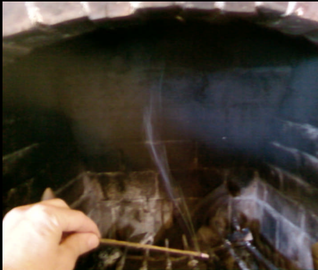
The fireplace chimney
