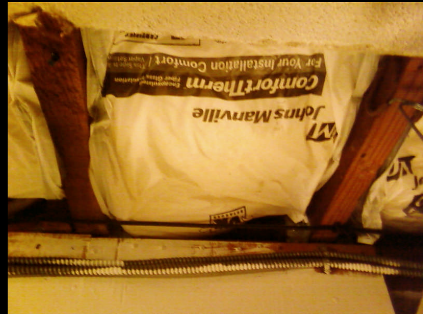
Under the floor above the garage
