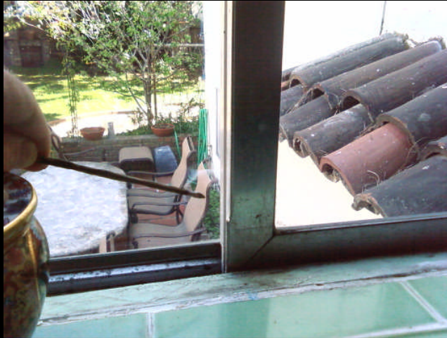
Old aluminum frame, single-pane window
