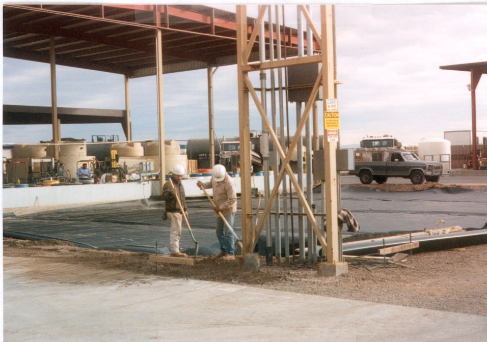
Final preparations on liner prior to covering
