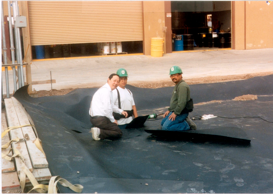
Sump area for liner being installed
