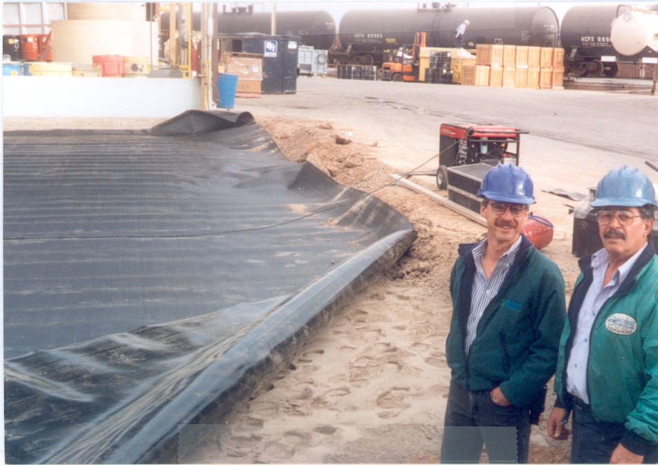
Liner being unrolled under tank farm
