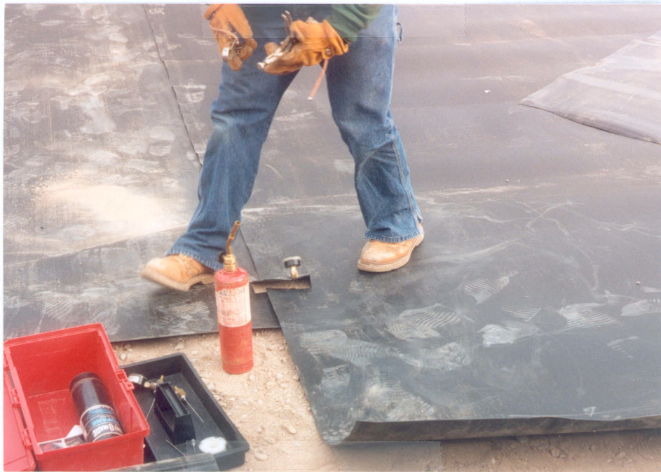
Liner seal being tested for leaks
