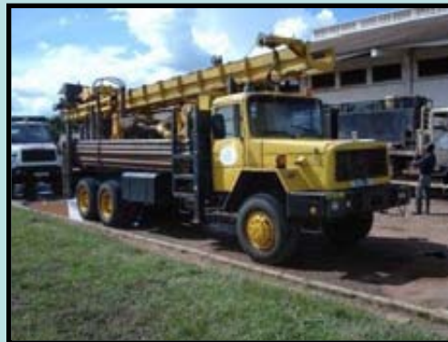
Materials to Site
