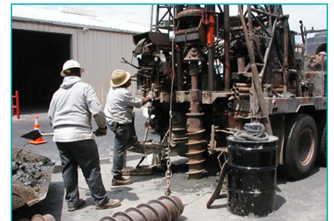
Installation of a monitoring well at Romic.
