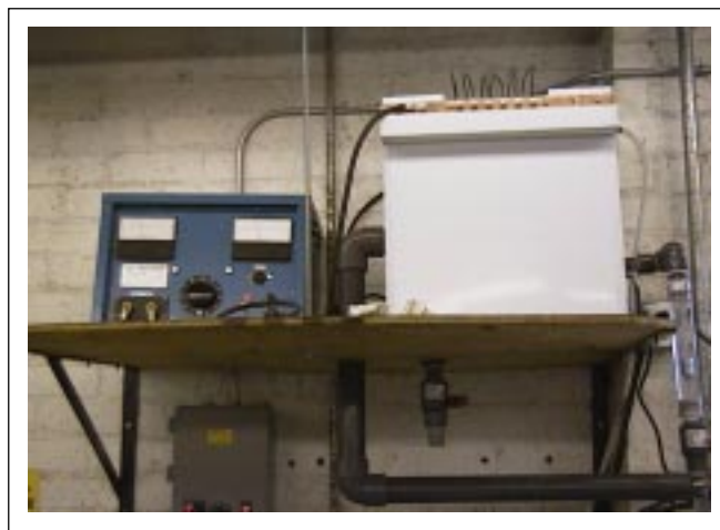
Figure 1. Electrowinning Rectifier and Electrolytic Cell
