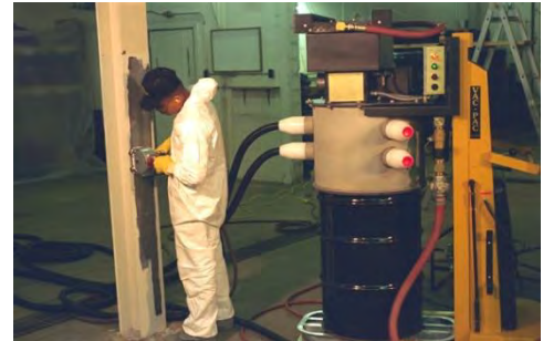
Worker is using the roto-peen (scabblers) attachment; VAC-PAC collection system shown with 55 gal drum.
