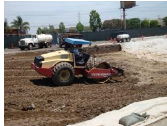
Compacting Soil under treatment pad area (5/21/2013)
