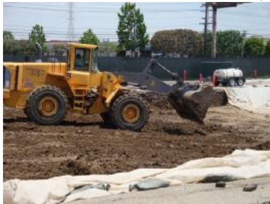
Placing backfill in treatment pad area prior to compaction (5/21/2013)
