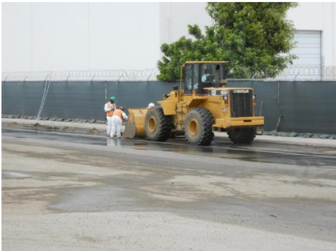
Figure 26: Workers cleaning up along newly installed realigned trench
