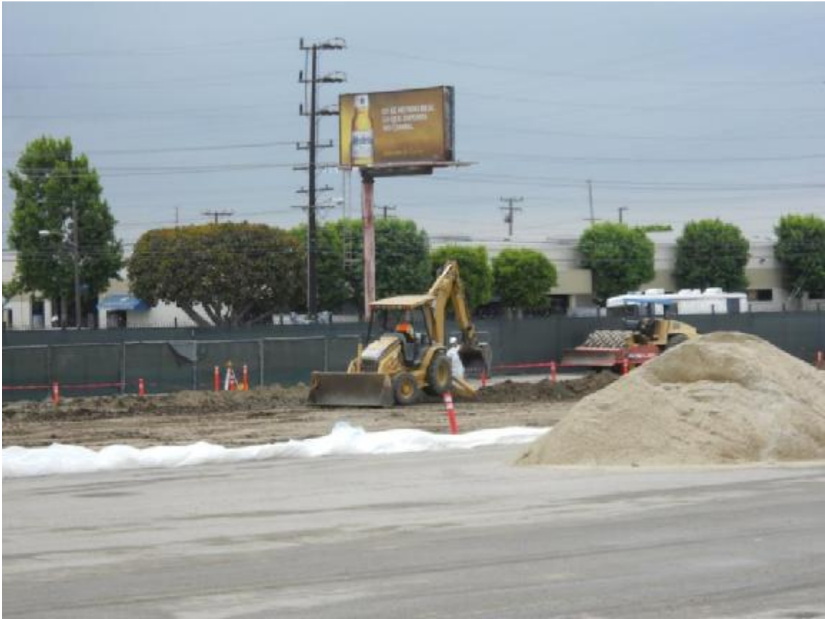
Figure 17: Montrose site trenching in progress
