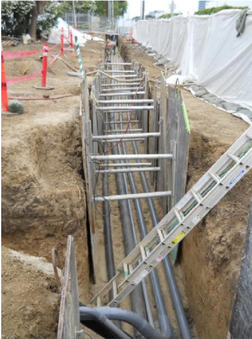
Figure 4: Pipes in trench with shoring
