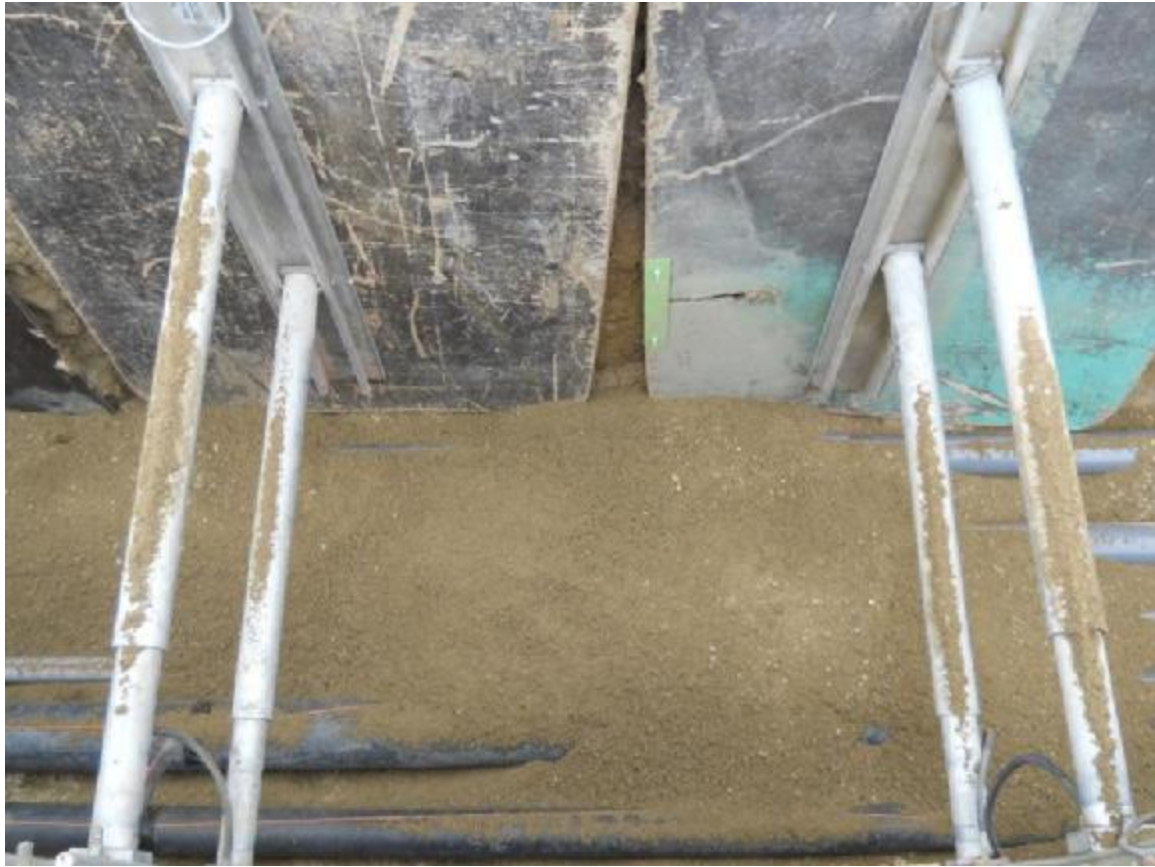
Figure 14: Trench with some sand backfill
