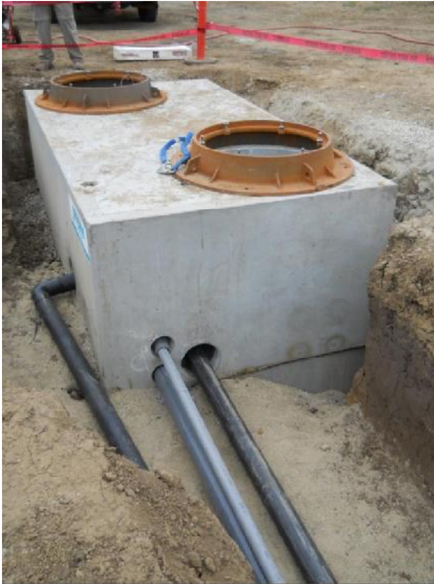
Figure 11: Precast vault that contained the pressure gauges
