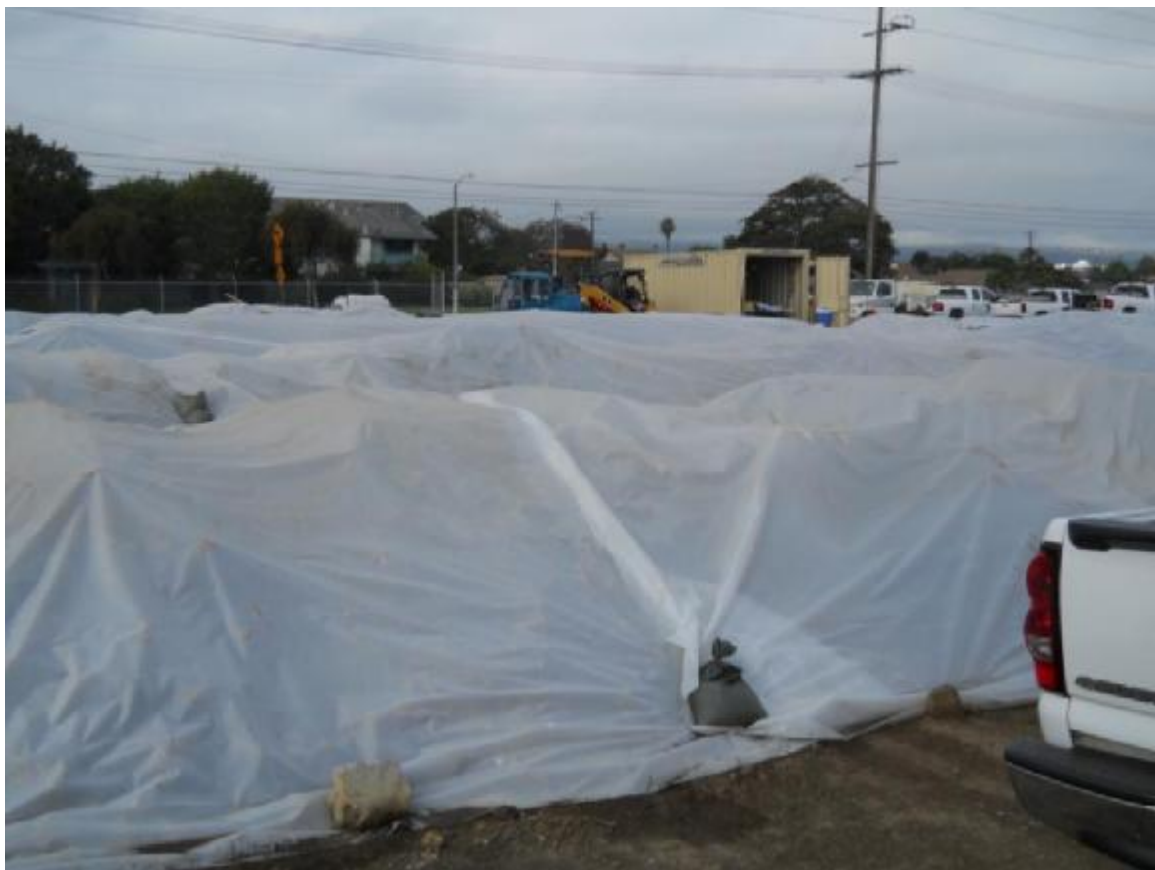
Figure 1: Covered stock piles at Waste Management site.
