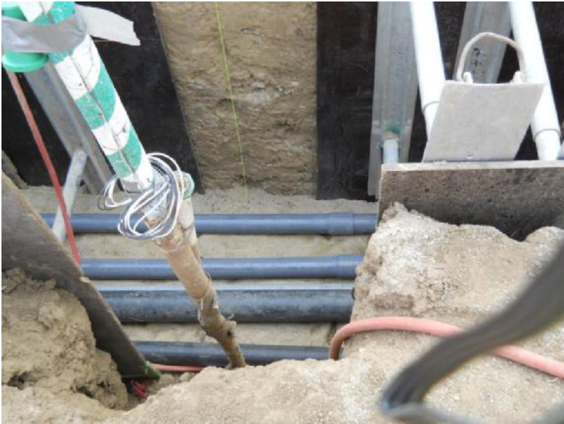
Figure 3: Close-up view of pipes in trench with shoring
