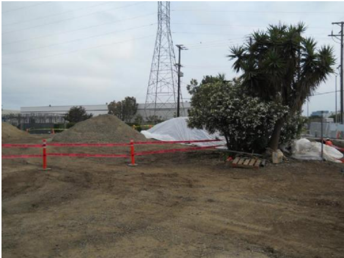
Figure 7: Gravel stockpile and covered soil stockpile
