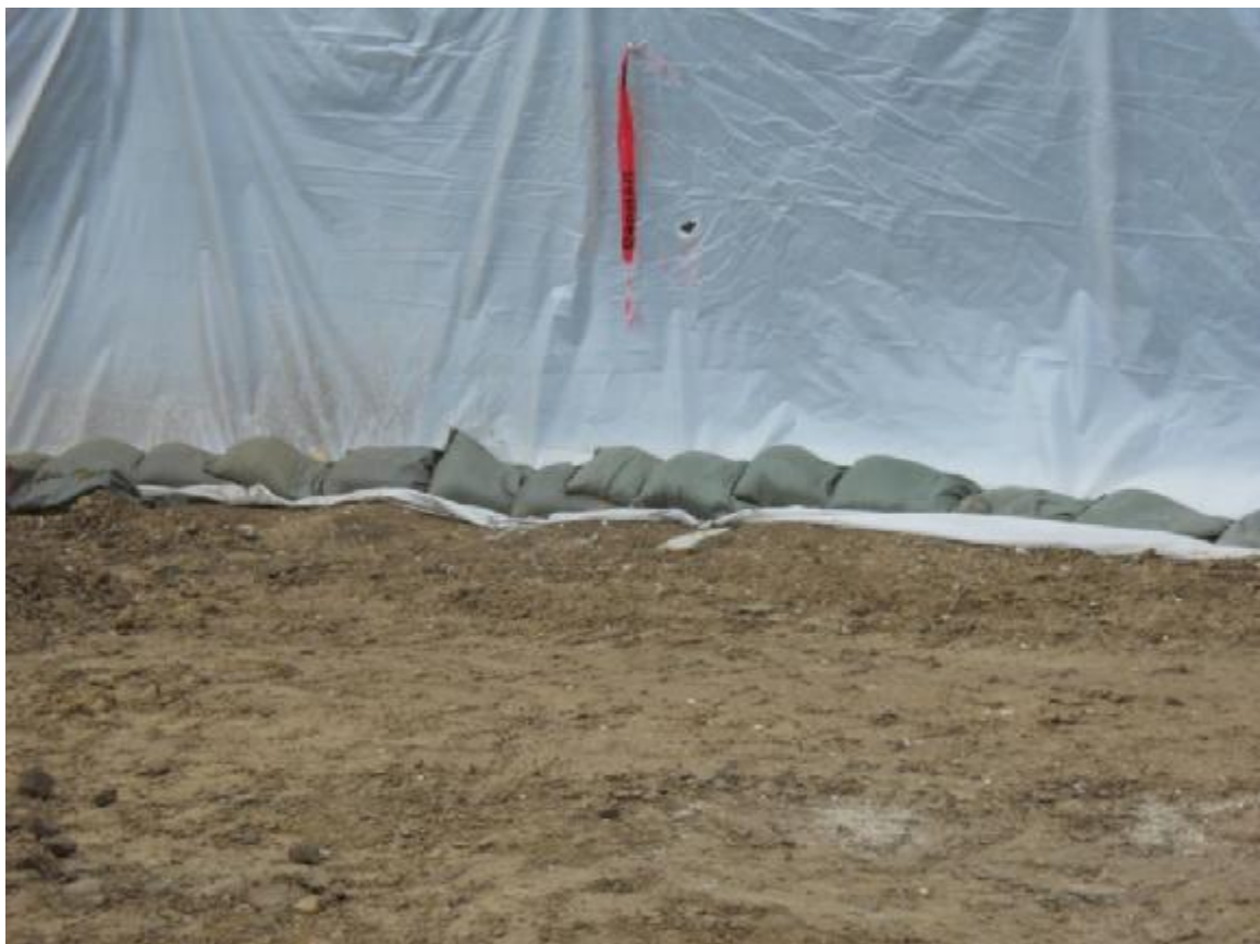
Figure 8: Property line fence with plastic to prevent dust migration
