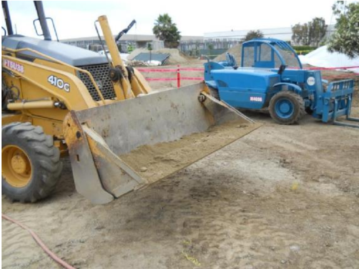
Figure 15: Loader with bucket of sand to begin backfill
