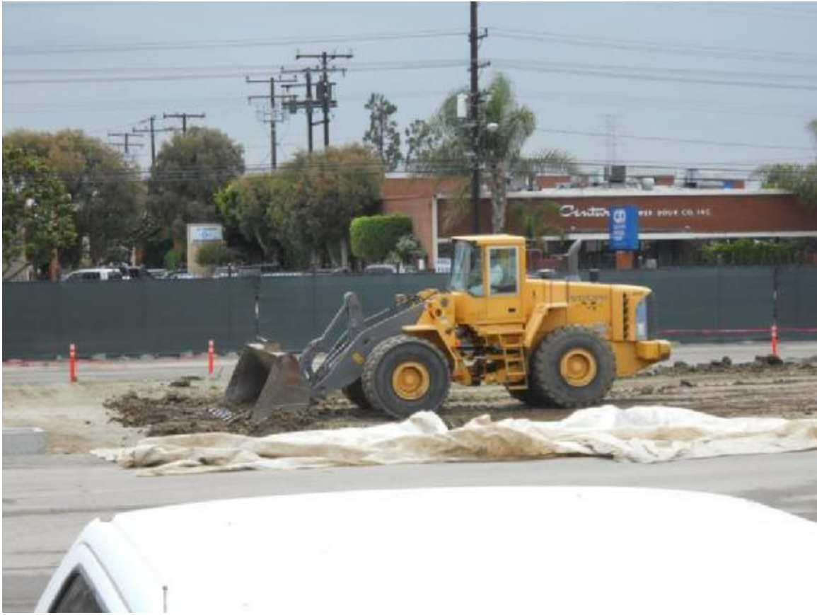
Figure 16: Montrose site grading in progress
