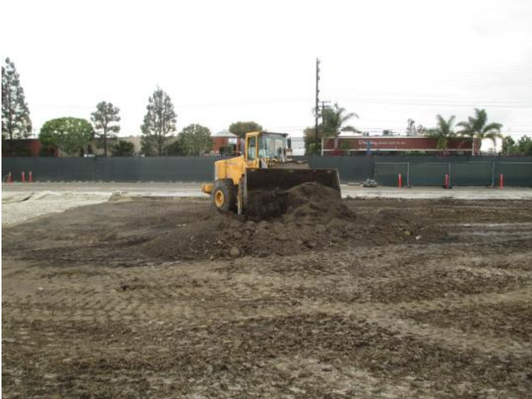
Figure 1: crushed asphalt and soil piles ready for mixing (top). Asphalt and soil being mixed by front loader, and well blended prior to being placed in fill layers (bottom).
