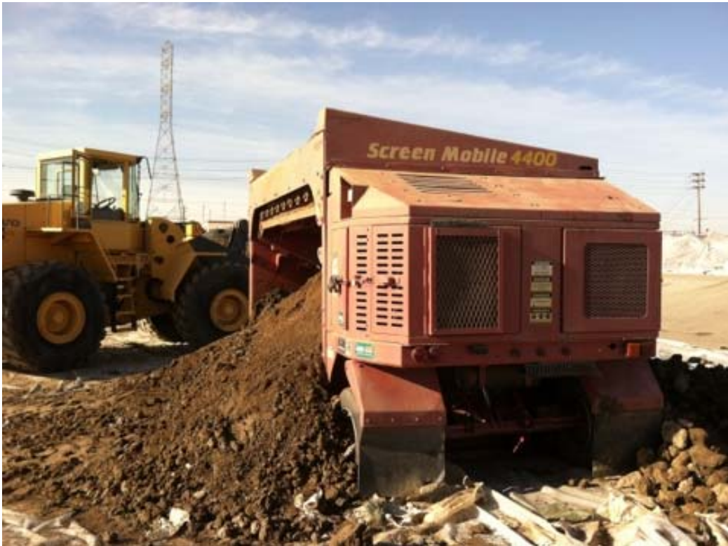
Figure 2: Soil screening machine.
