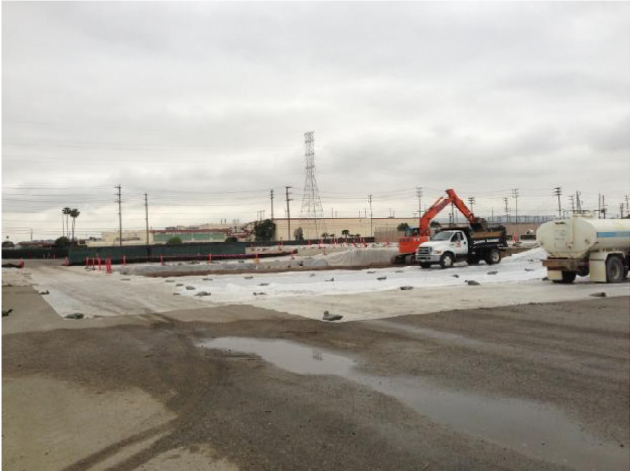
Excavation area. Taken facing southwest.
