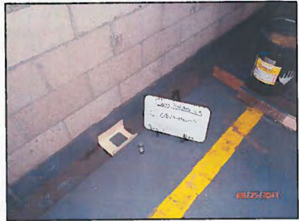
Photo 8: Wipe Sample in Dirty Gutter in Bay 3
