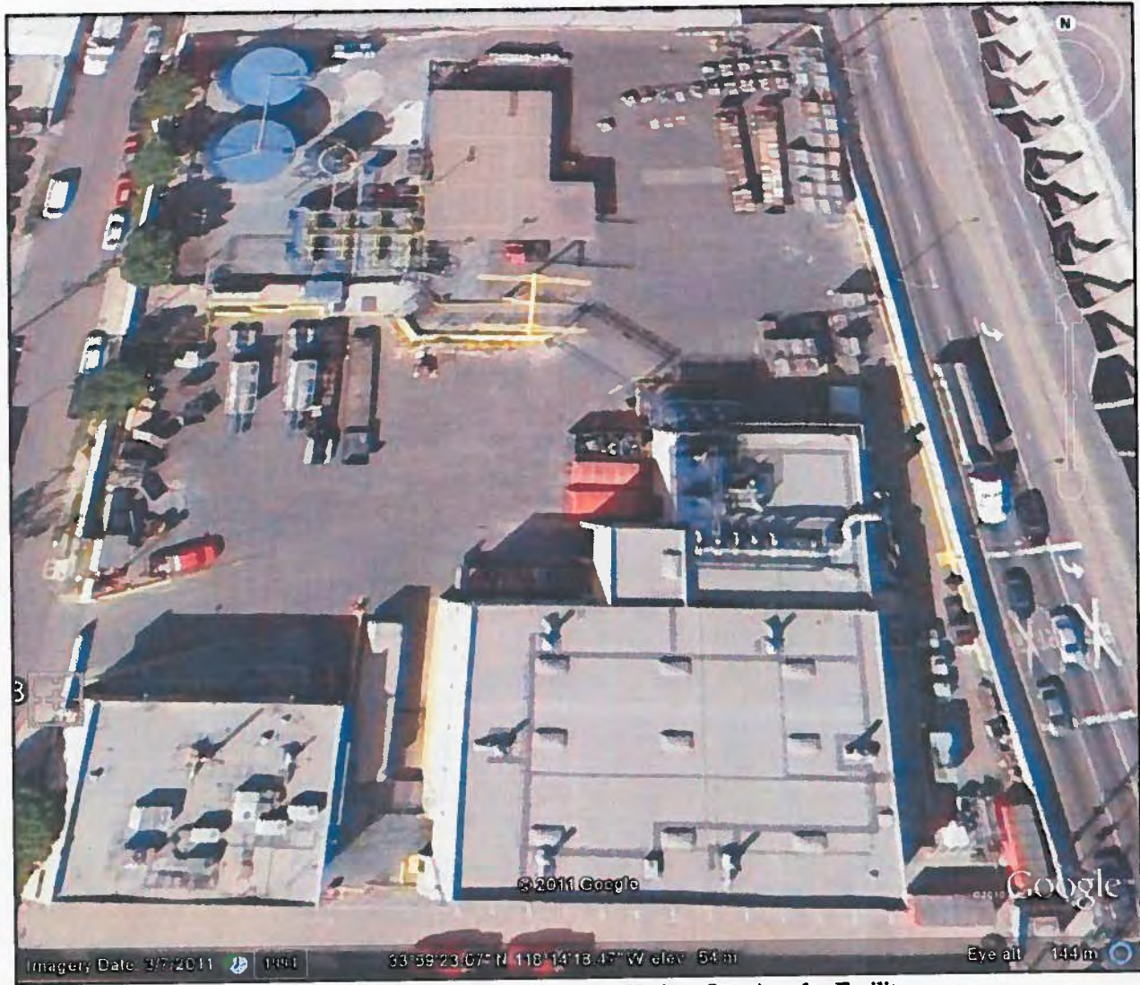
Google Earth Aerial View of the Clean Harbors Los Angeles Facility
