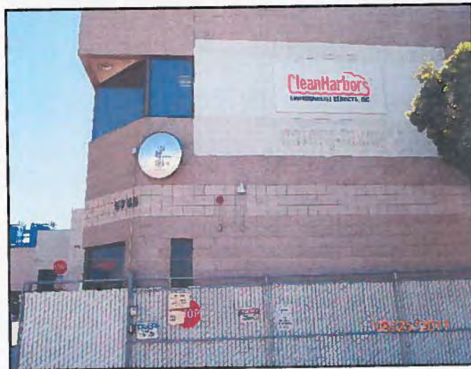
Photo 1 - Entrance to the Facility
