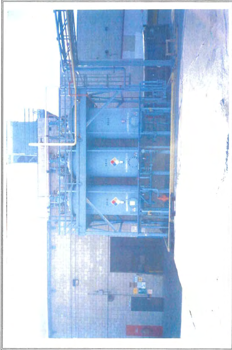
Photo 3 : View of 3,000 Gal Oil Storage Tanks.
