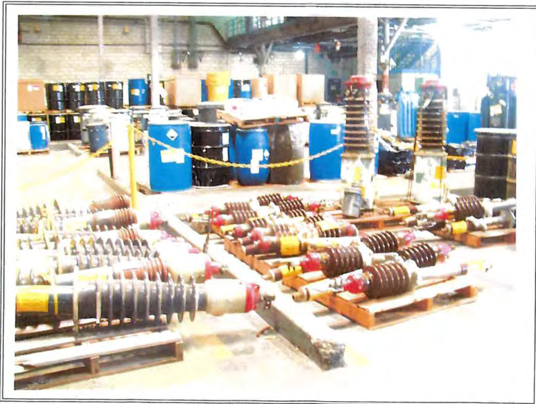
Photo 13 : View of more bushings inside CHI "Container Storage Warehouse."
