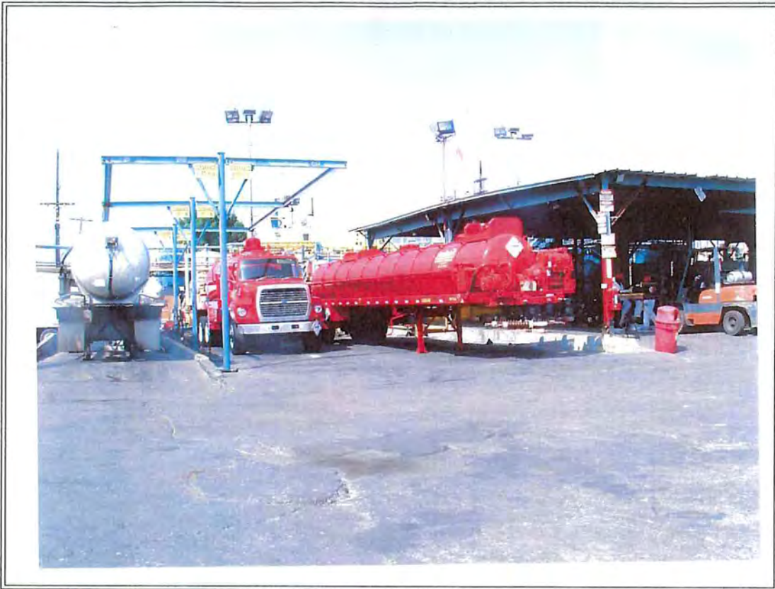
Photo 4 : View of yard showing tanker unloading facility.
