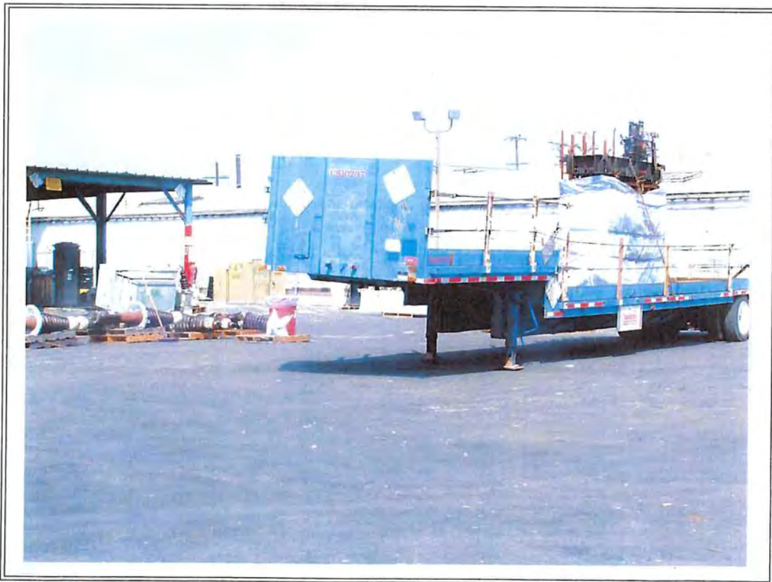
Photo 9 : View of plastic wrapped transformers on trailer & more stored bushings at left.
