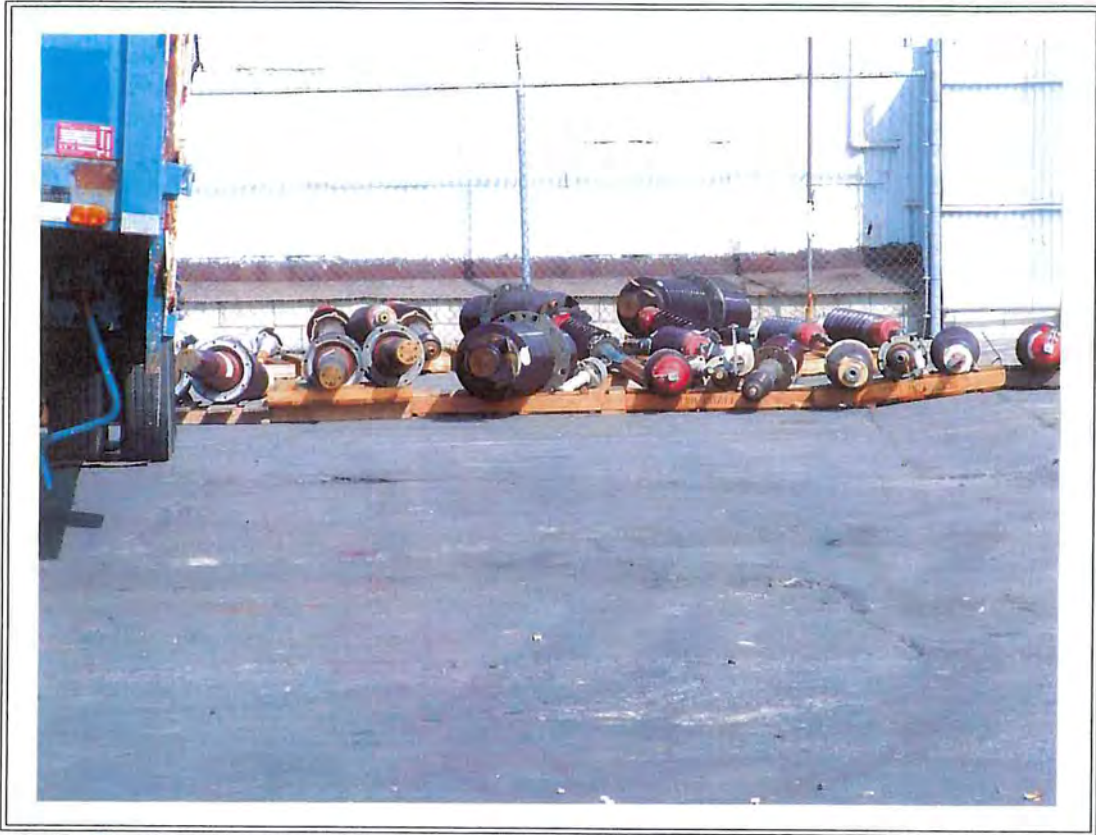
Photo 8 : View of transformer bushings stored along fence line.
