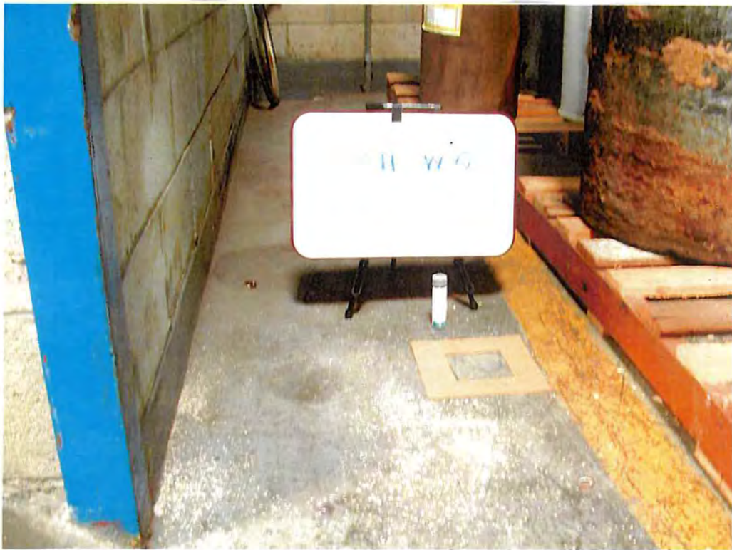
Photo 22 :View of wipe sample #6 collected inside PCB storage bay.
