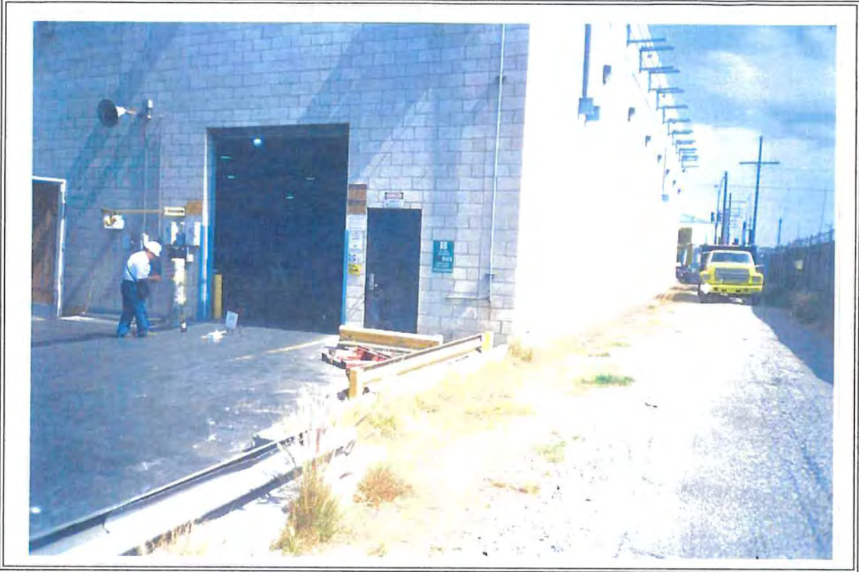
Photo 2 : View of ATSF Rail Right-of-Way Between CHI Storage & Slauson Ave.
