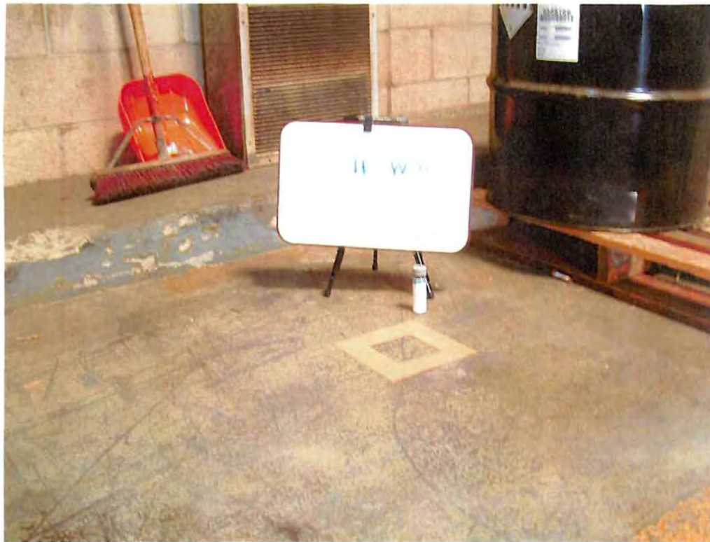
Photo 23 :View of wipe sample #8 collected inside PCB storage bay.
