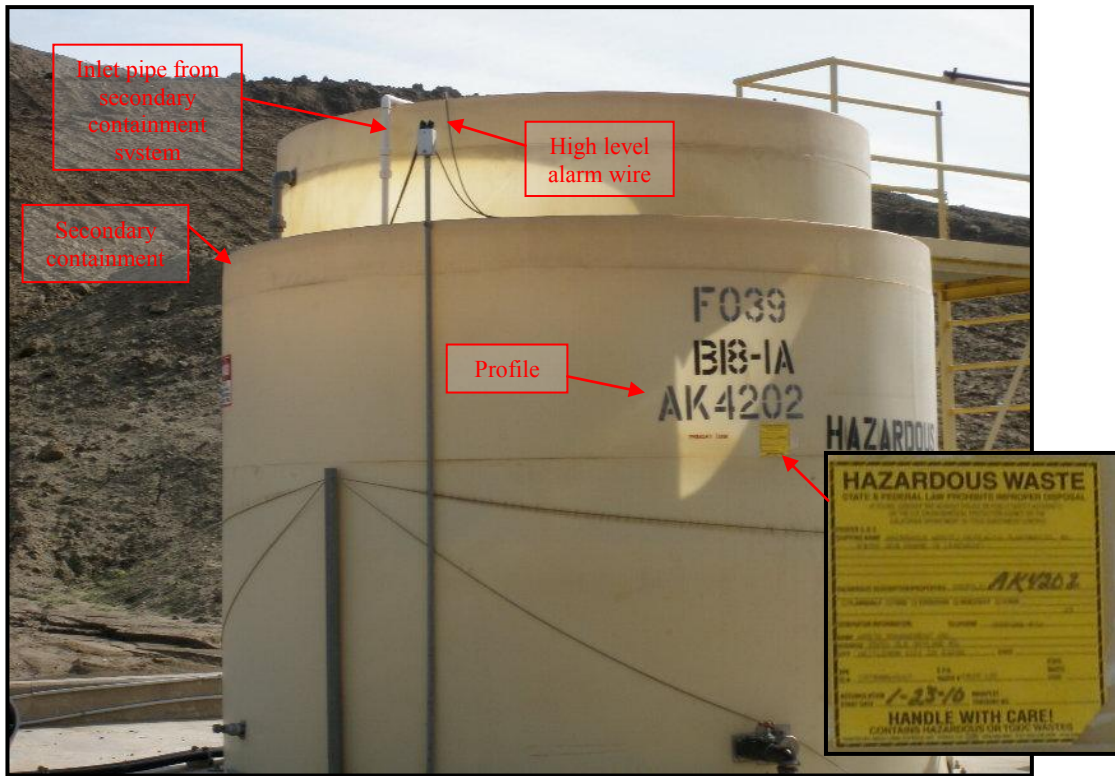
B-18 Phase 1A leachate collection tank
