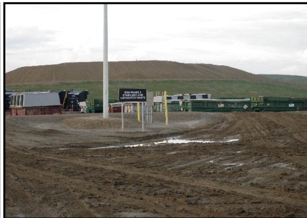
BSU Phase 2 (facing north)
