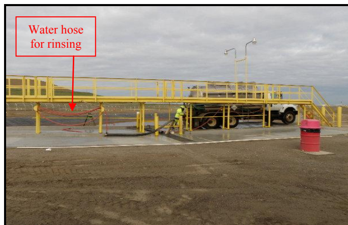
P-9 Unloading Area (facing east)
