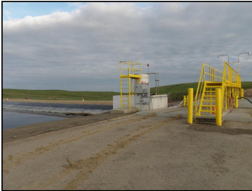
P-16: Leachate collection tank and unloading area (facing south)
