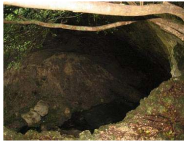
Hilton Hotel Sinkhole
