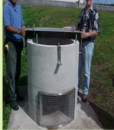
Bored or Drilled UIC Wells with Screen Above Grade
