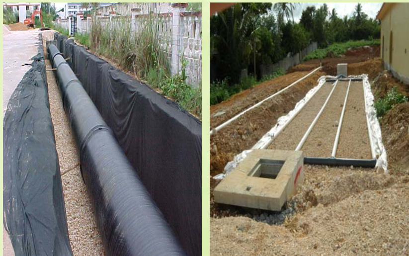
UIC System with Perforated Pipe
