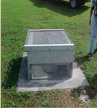
Bored or Drilled UIC Wells with Screen Above Grade
