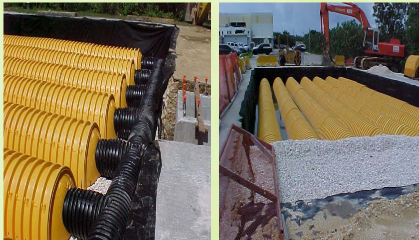
UIC System with Chambers
