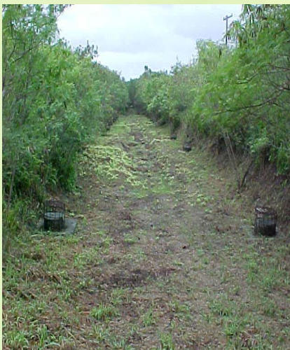
Bored or Drilled UIC Wells within a Ponding Basin
