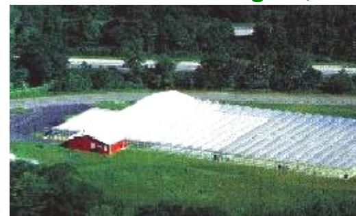
Greenhouse Burlington, NJ
