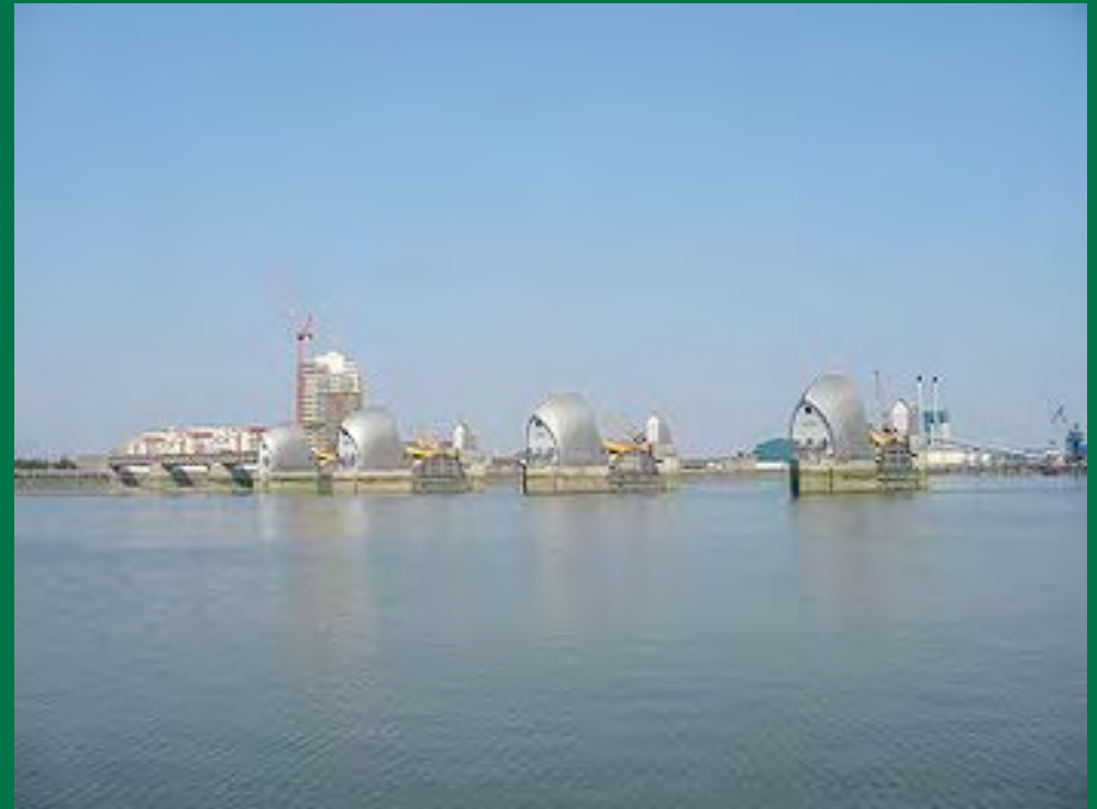
Aerial view of the Thames Barrier with all gates up from the bottom of the river to staunch the flow of the water in the river. Source: http://www.the-river-thames.co.uk/weather.htm ; accessed January 5, 2006.
