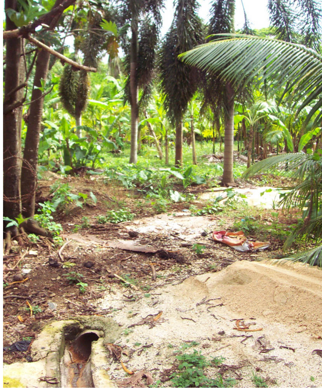
Effluent Drainage to Field
