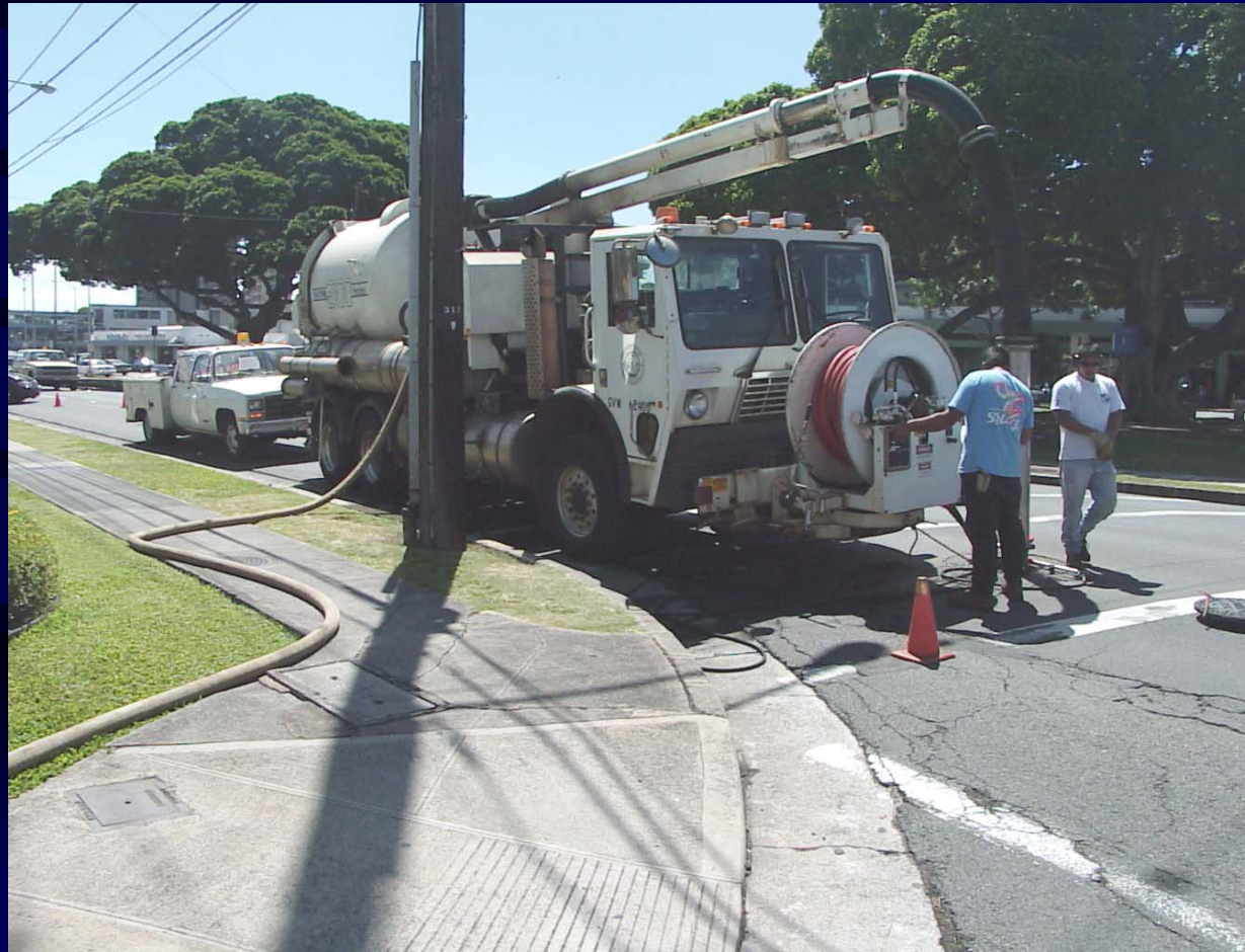
Storm drain maintenance with vactor trucks
