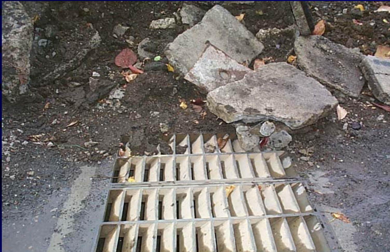
Storm Drain Protection
