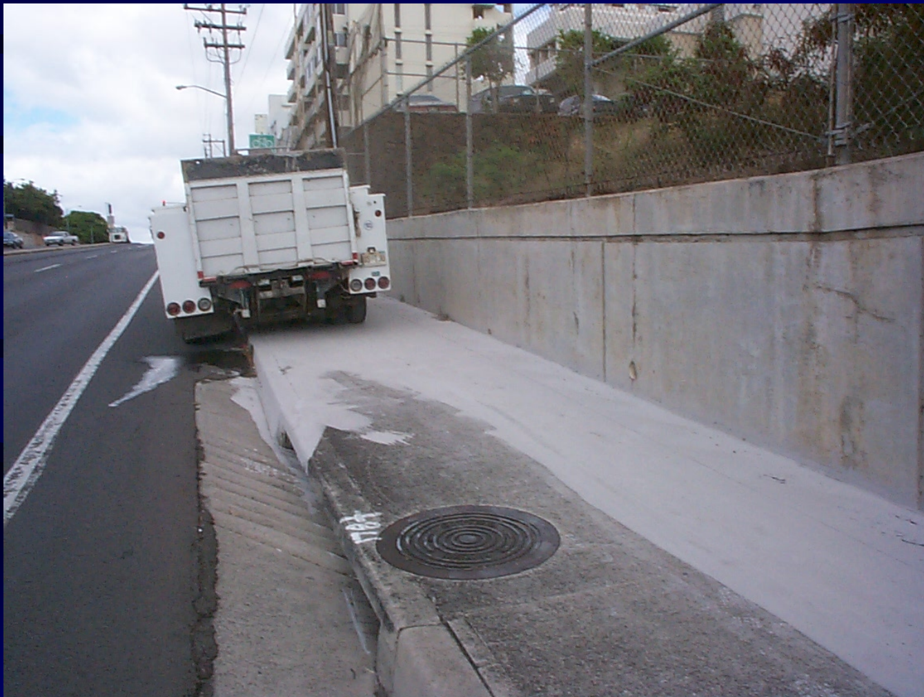
Storm Drain Protection
