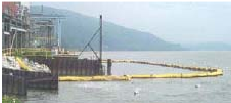
Figure 4.16 Gunderboom® MLEST™ Deployed at Lovett Generating Station
