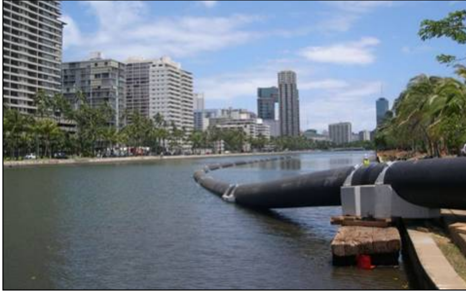
Photo 1: Installation of 42-inch-diameter HDPE Pipeline (courtesy: City and County of Honolulu)
