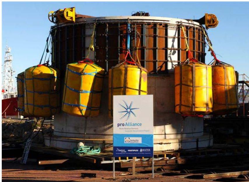
Figure 8-2: Velocity Cap for the 38 MGD Perth Australia Seawater Desalination Facility
