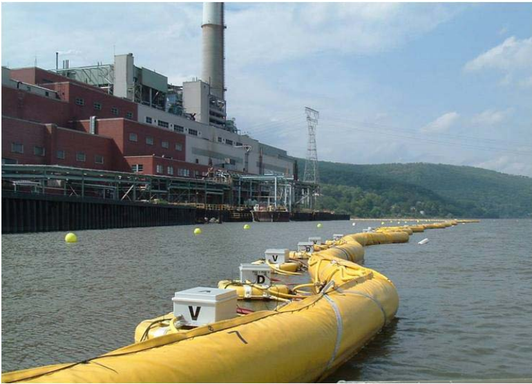
Figure 8-7: An Aquatic Filter Barrier Screen
