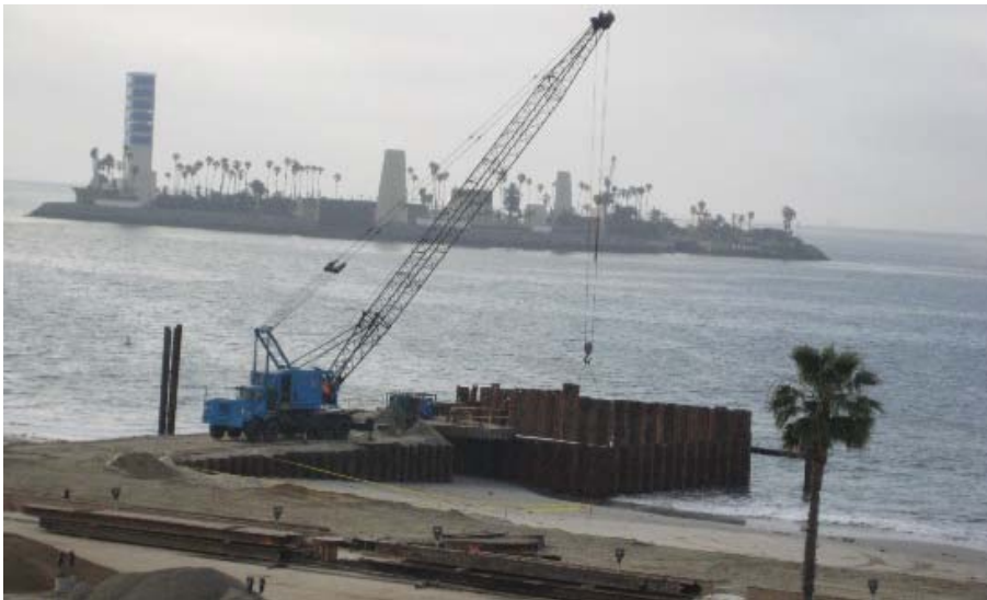
Figure 3-7: Excavation of a Pilot-Scale Engineered Beach Infiltration Gallery, Long Beach, CA (LBWD, 2008)
