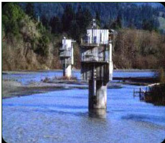
Figure 3-5: Horizontal Collector Wells in the Mad River, Eureka, California
