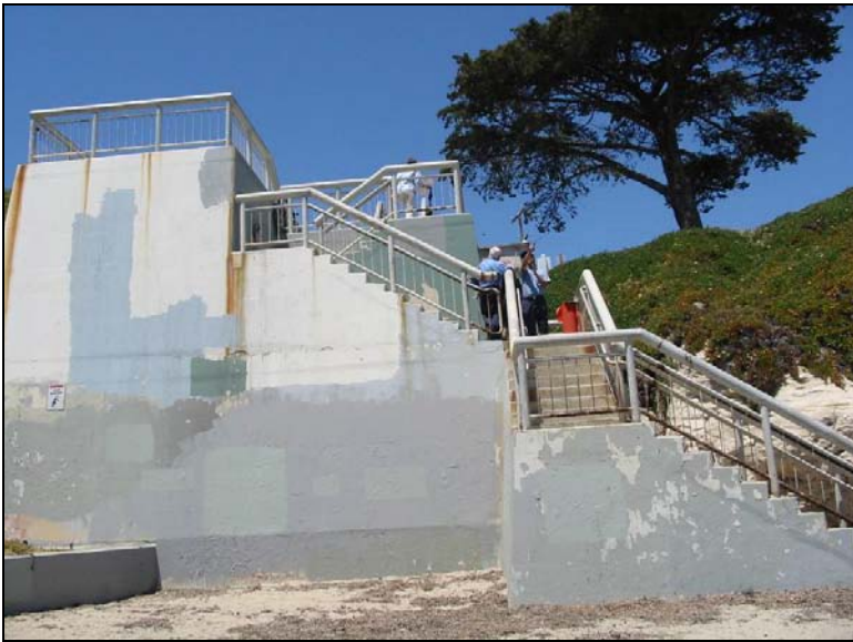
Figure 10-5: Existing Outfall Junction Structure
