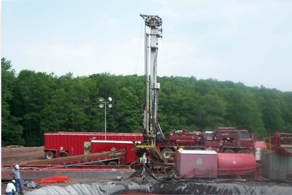
Topset rig drilling surface- and intermediate-cased intervals
