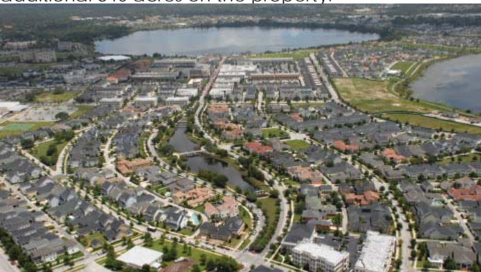
Aerial view of the Baldwin Park redevelopment project.
