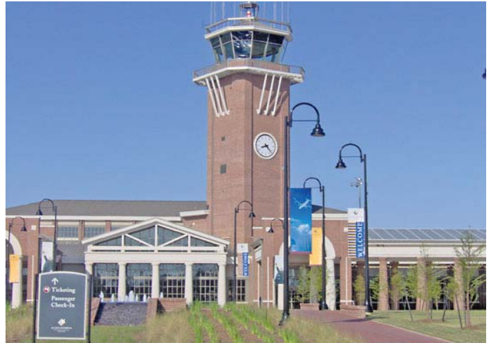
Control tower at the Alexandria International Airport
