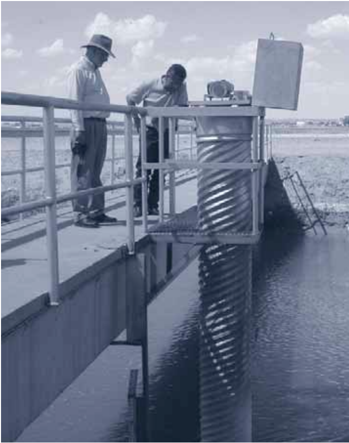
To promote water conservation by preventing over-delivery, this stage recorder monitors the water flow in an irrigation canal in the Rio Grande.
