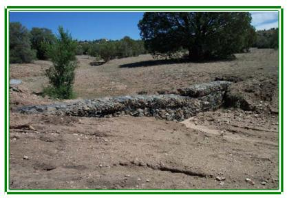
Yavapai-Prescott Indian Tribe protecting water quality by preventing erosion with a gabion structure in an eroded drainage area.
