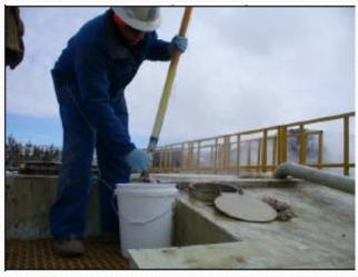
Collecting flowback sample from frac tanks using a bailer
