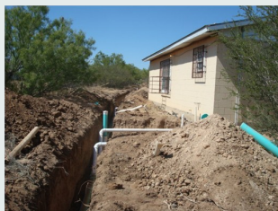
Construction of water infrastructure hookups to homes
